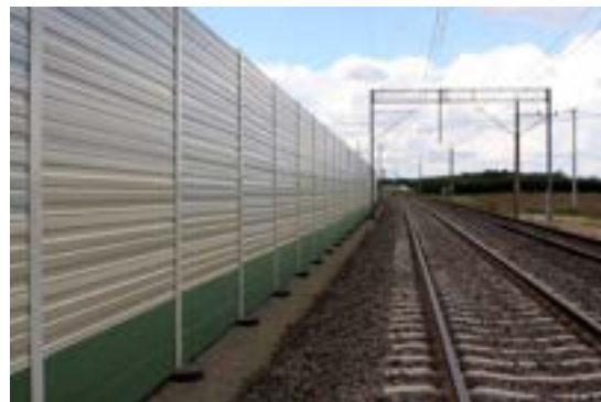
Installed aluminium sound barrier
