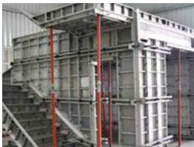
Aluminium formwork for concrete work
