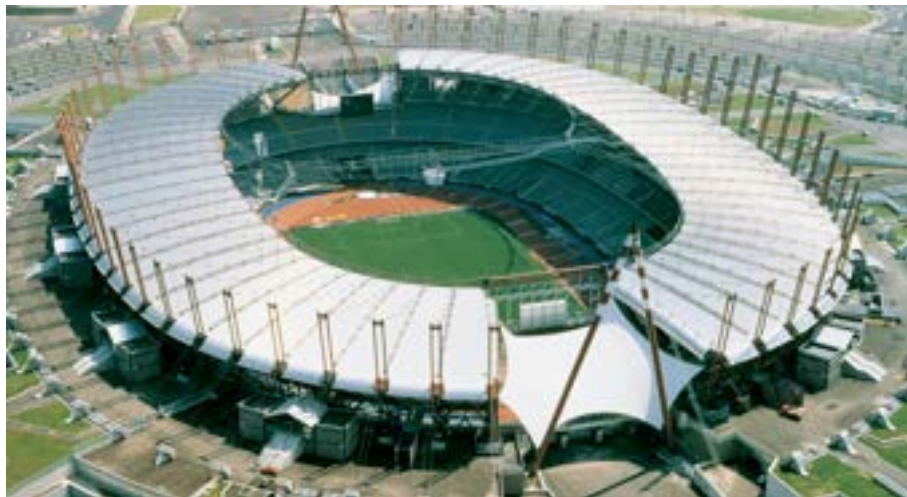
Wide-span structure of a stadium with visible steel beams, structural elements, and aluminium panels.
