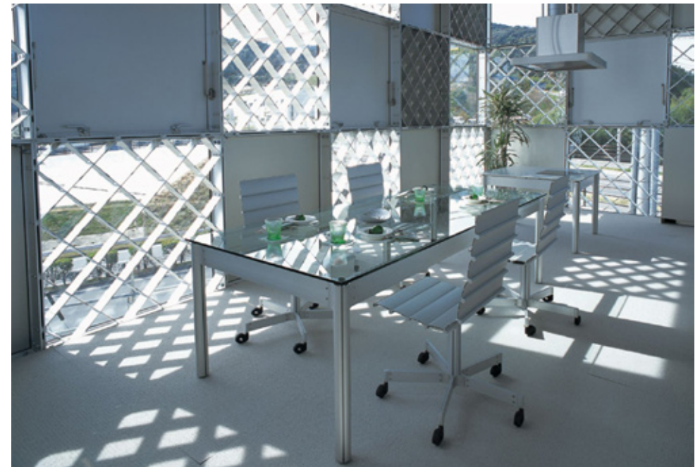
Fig 3.8 Extruded aluminium structure and solar shading of the Aluminium House System, Kyushu, Japan, architect Riken Yamamoto & Fieldshop
