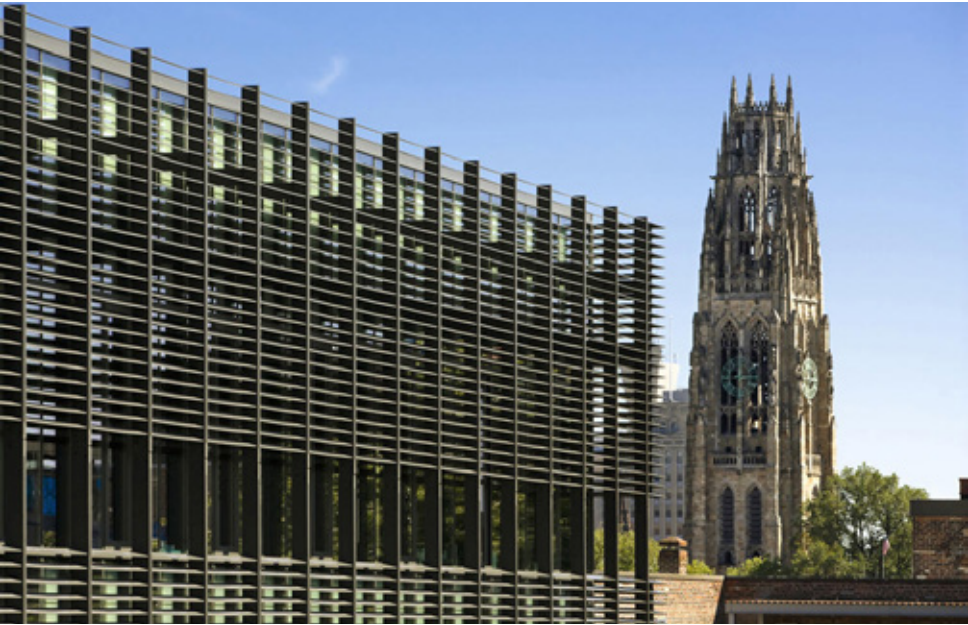
Fig 3.9 Bespoke extruded aluminium solar shading for Yale Sculpture Building and Gallery, designed by KieranTimberlake in collaboration with Schüco, completed in 2007
