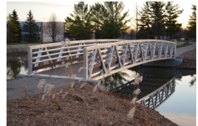
Fig 2.6 Welded aluminium pedestrian bridge by MAADI Group
