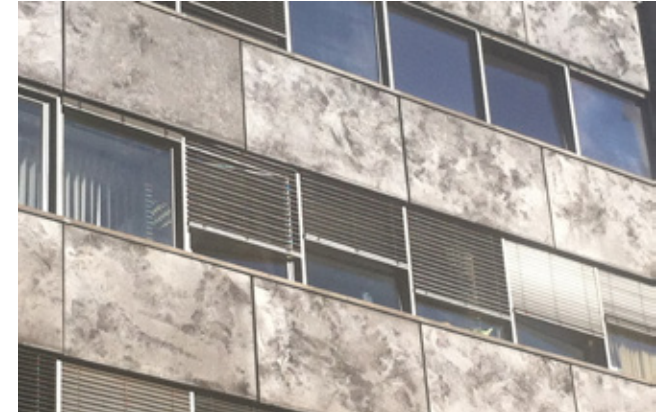
Fig 2.15 The Ljubljana Television Centre, Slovenia, used horizontally cast aluminium cladding panels in 1974, architect France Rihtar in collaboration with Branko Kraševac
