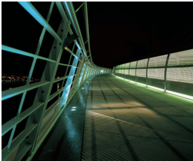
Fig 5.151 The ribbed aluminium bridge deck of the cycle lane of the Millennium Bridge, Gateshead
