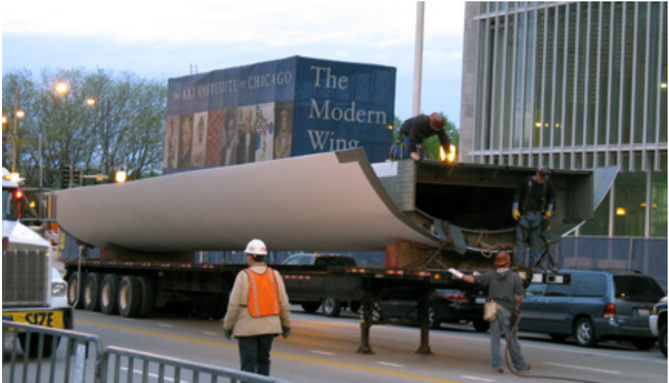
Fig 5.160 Transporting the large prefabricated sections of Nichols Bridgeway
