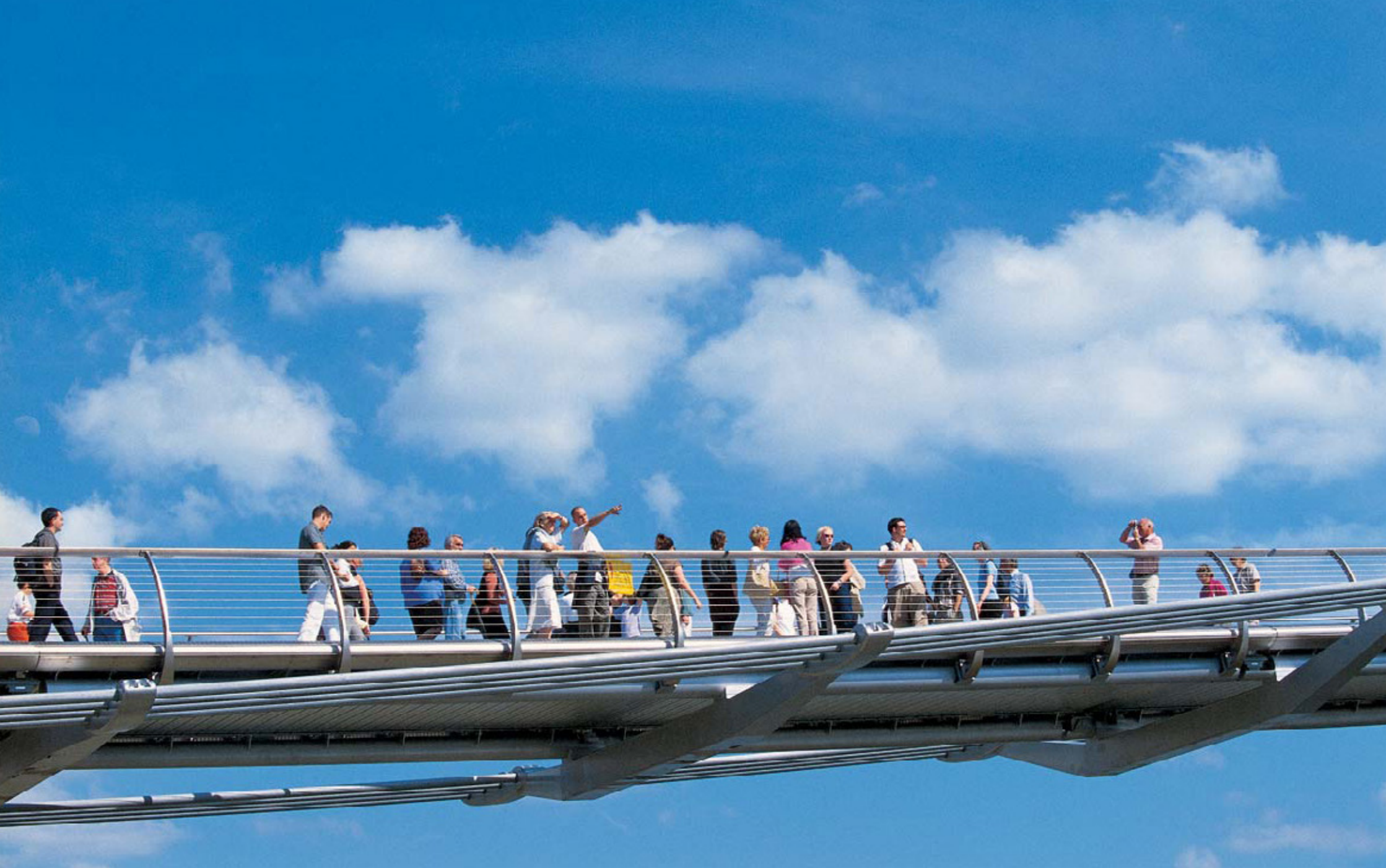
Fig 5.130 The low slung suspension cables of the Millennium Bridge, London, create an effortless openness to view and be viewed
