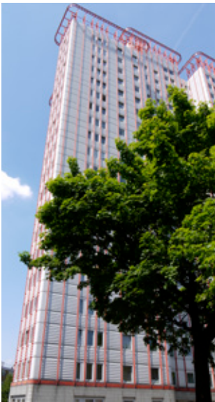
Fig 4.1 The overcladding of Parsons House is a system of polyester powder coated aluminium panels and windows with articulated mullions designed by Peter Bell & Partners, 1986
