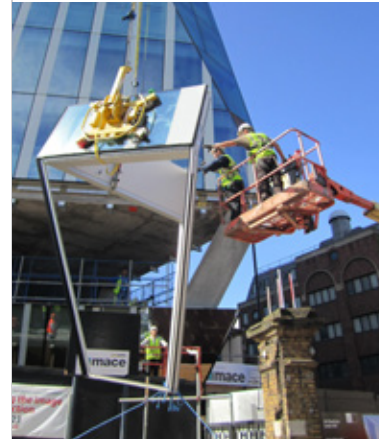
Fig 7.24 Installation of the unitised aluminium curtain walling of 240 Blackfriars Road fabricated by Scheldebouw
