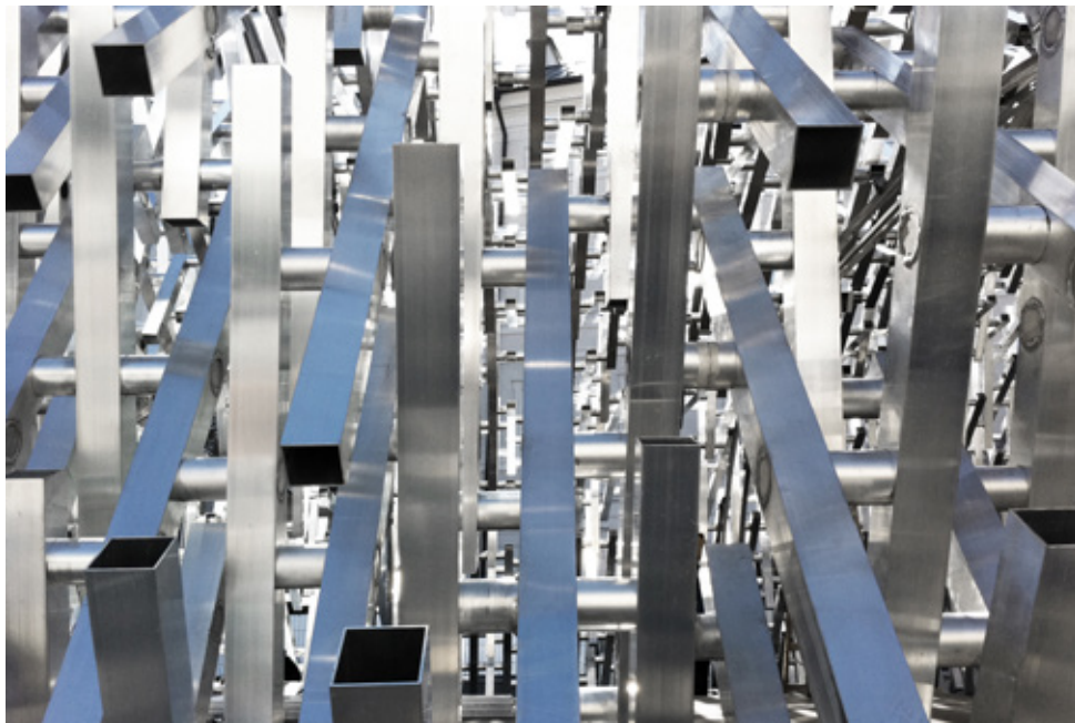
Fig 5.222 An aggregated aluminium structure formed of standard extrusions
