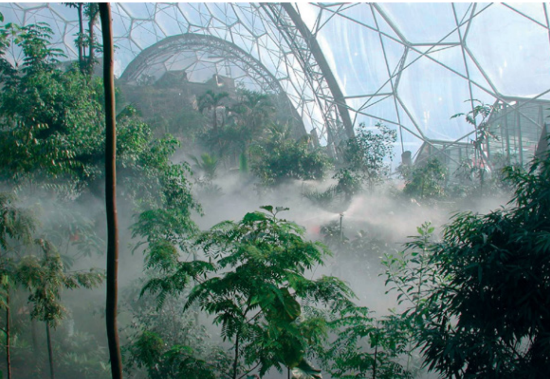
Fig 6.28 The rainforest Biome sheltered by the lightweight ETFE pillows
