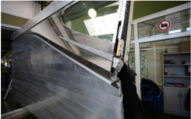
Fig 4.34 Sky window — cladding interface of the 10 Hills Place prototype
