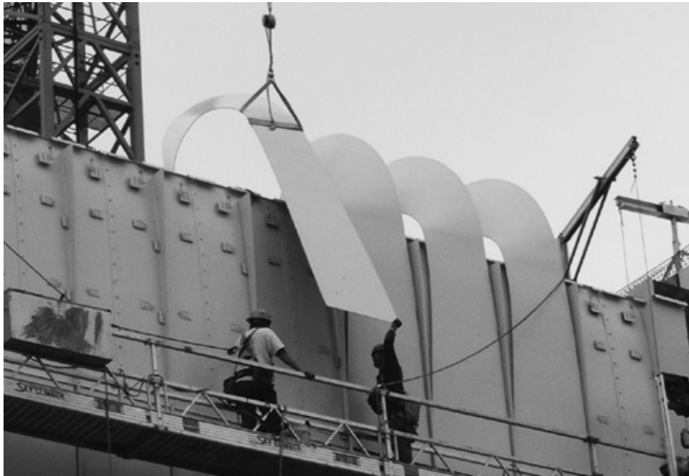
Fig 3.52 The fixing sequence of cowl-panels
