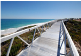
Fig 5.95 Aluminium deck of Yanchep Bridge, designed and fabricated by Peter Maier Leichtbau
