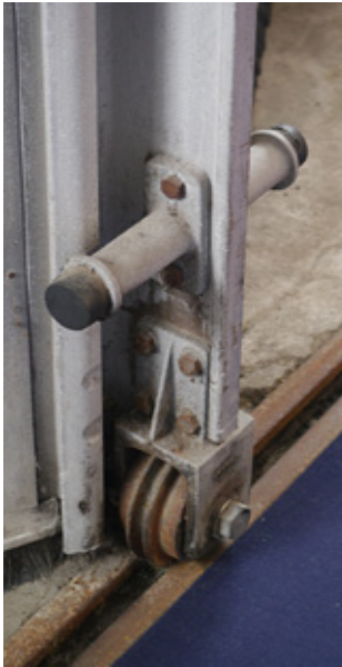
Fig 5.24 Steel bolts, steel wheels and steel track, fixing, supporting and guiding the aluminium Esavian doors, photographed 2016
