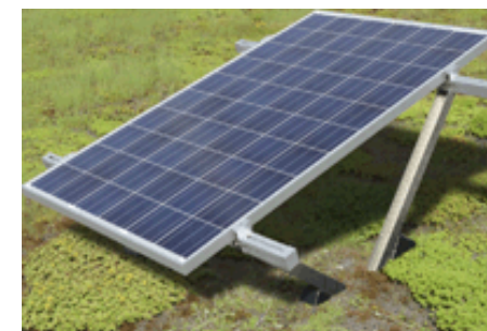
Fig 8.2 The photovoltaic panels are held above the extensive vegetation
