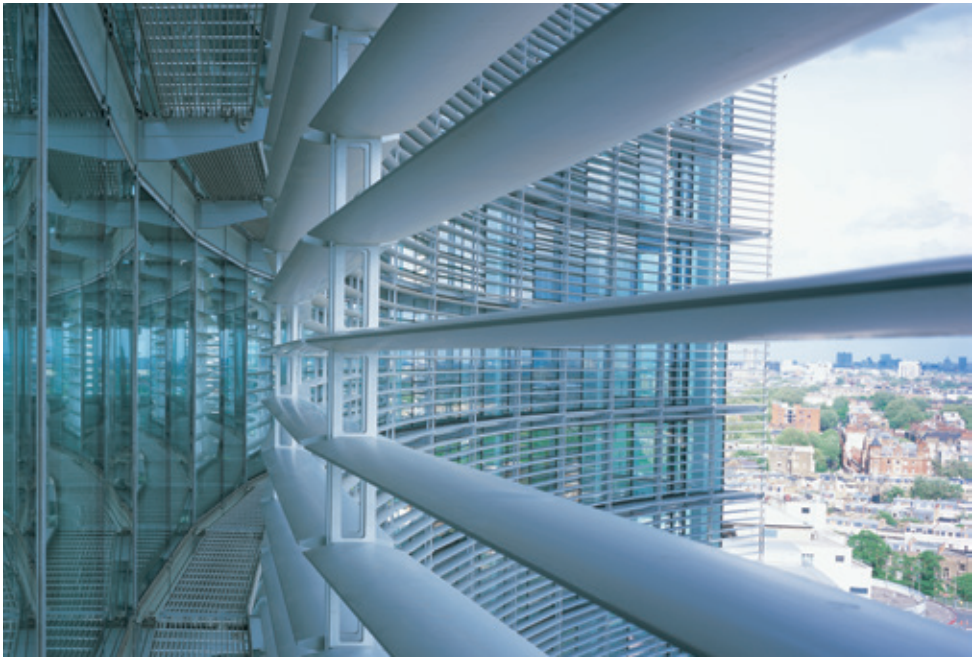
Fig 3.28 The gently faceted elliptical aluminium louvres of Empress State
