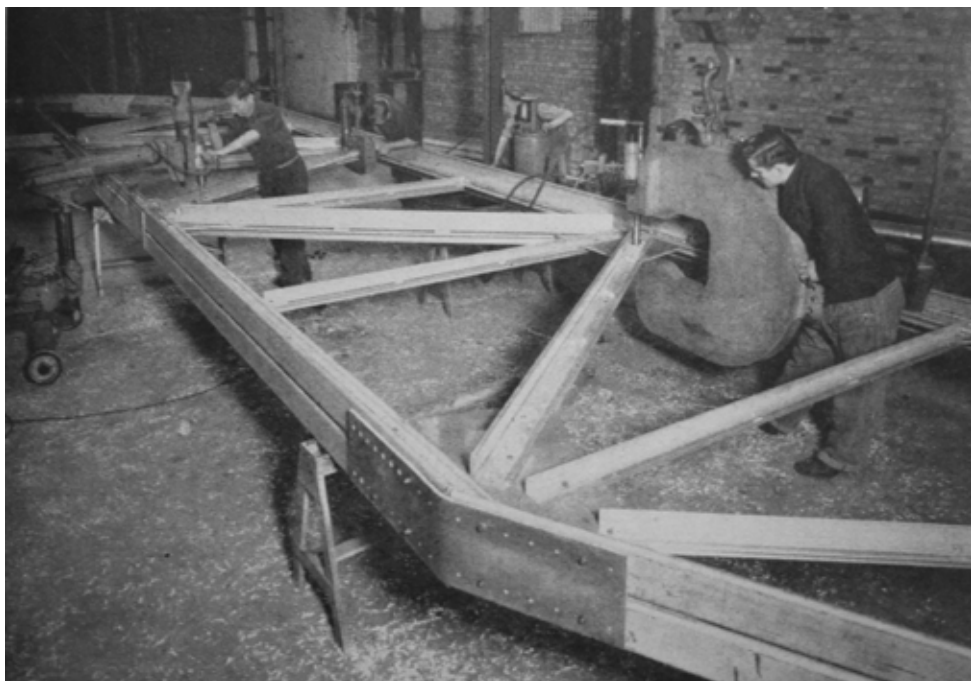
Fig 5.10 Cold riveting the aluminium trusses using a suspended ½ ton yoke
