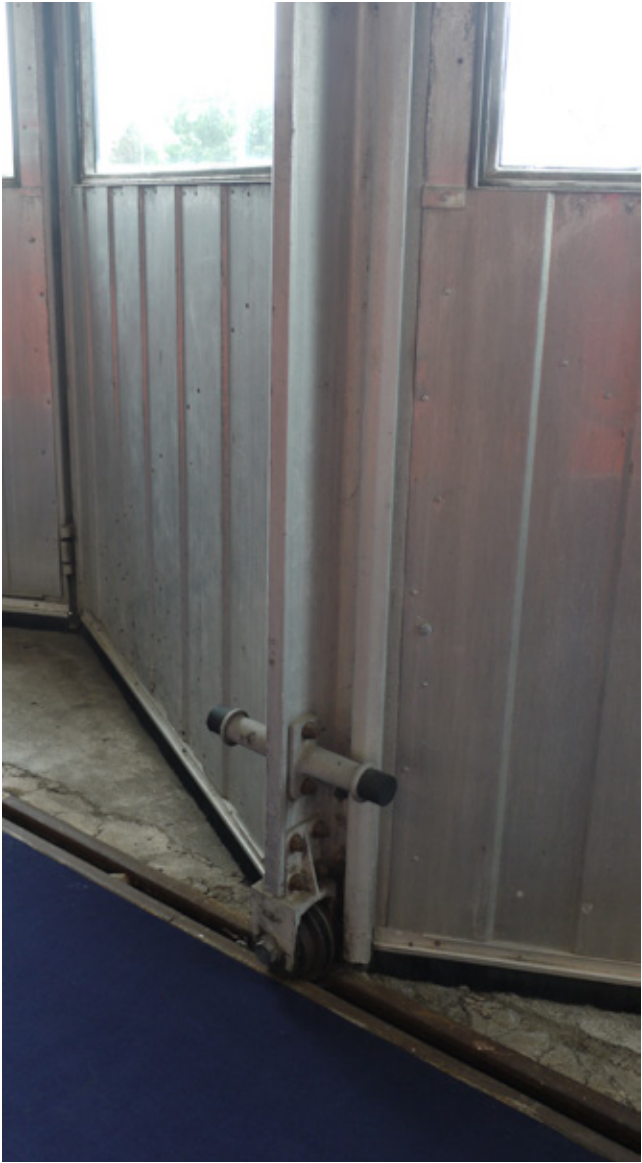
Fig 5.25 The hinge detail of the aluminium Esavian doors, underneath the vision panels of the north façade, photographed 2016
