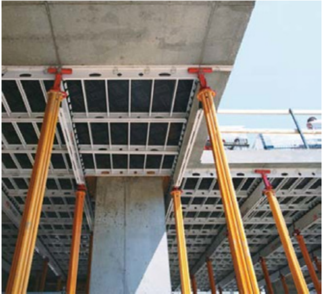
Fig 5.60 At the University Club Tower, Milwaukee, Wisconsin Aluminium formwork was assembled without a crane
