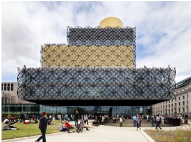
Fig 10.3 Library of Birmingham designed by Meccano Architekten for Birmingham City Council, shortlisted for the Stirling Prize in 2014, its building fabric includes silver and backmetallic polyester powder coated solar shading
