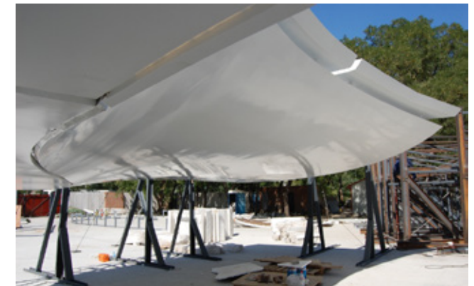
Fig 1.2 The 3mm polyester powder coated aluminium of the Soho Galaxy Prototype Zaha Hadid Architects fabricated by Permasteelisa
