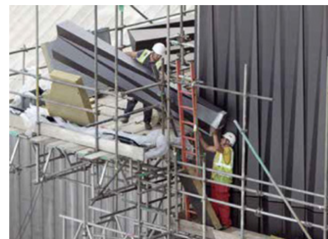
Fig 4.17 [right] Permasteelisa installing a folded aluminium rainscreen panel at Guy's Hospital Tower
