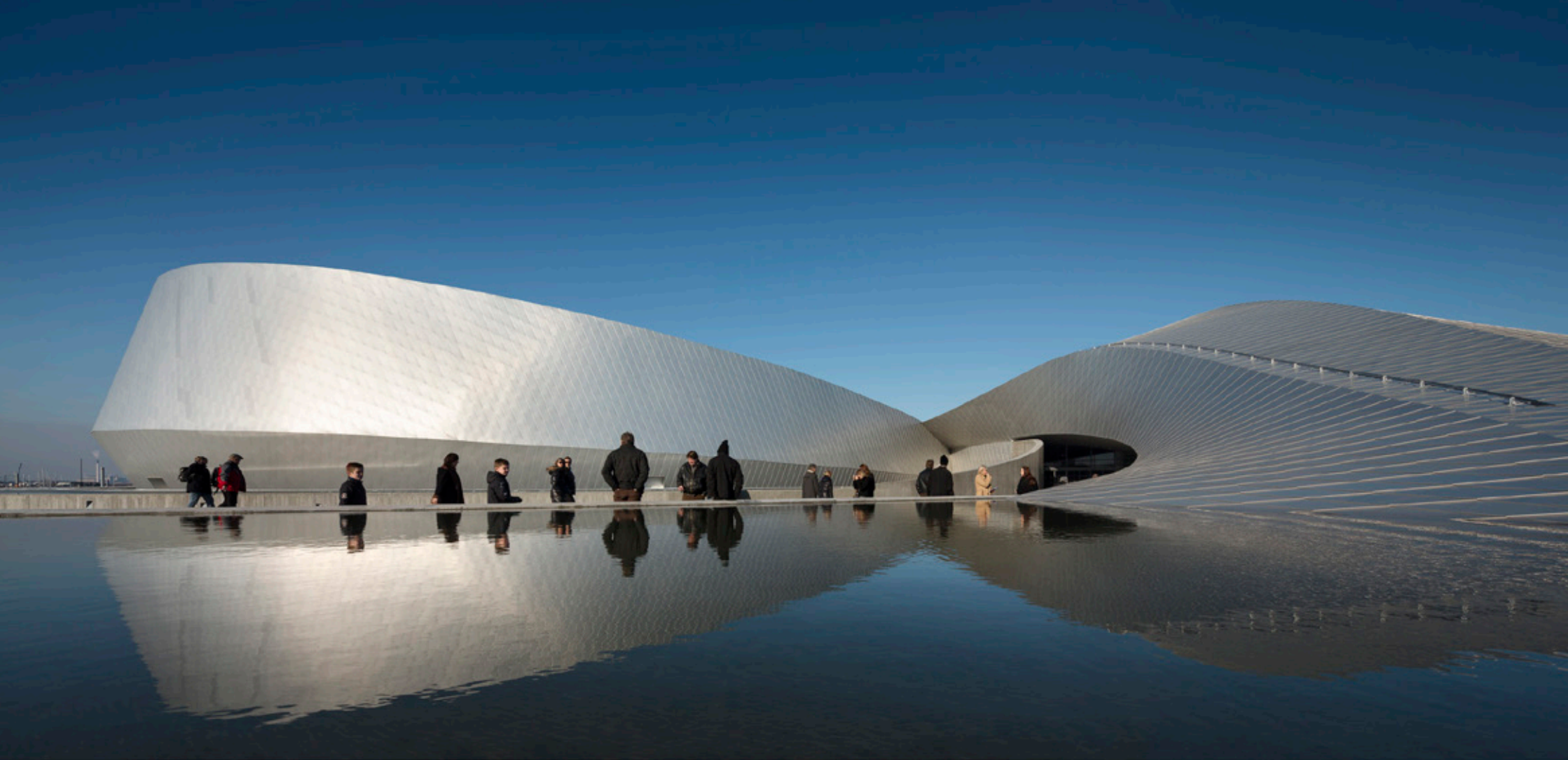
Fig 9.55 The shingled aluminium cladding dips into one of the reflective pools
