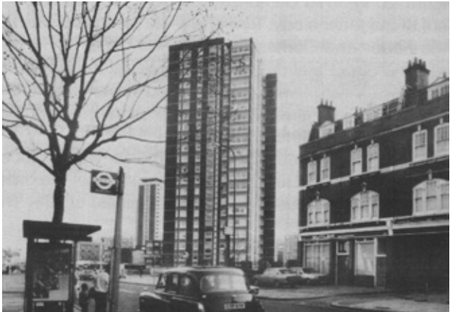
Fig 4.2 Parsons House completed in 1969 was constructed from brick, concrete frame and timber windows
