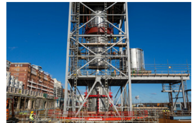
Fig 7.31 The jacking process of assembling the tower of the i360
