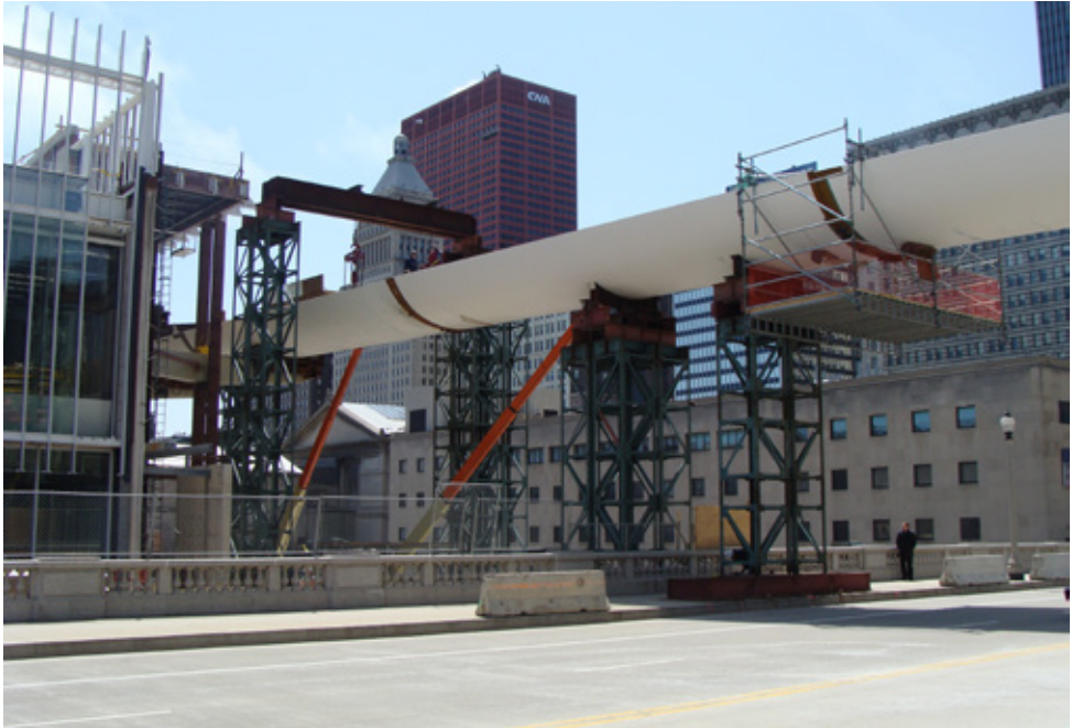
Fig 5.161 The assembly of Nichols Bridgeway from large prefabricated elements
