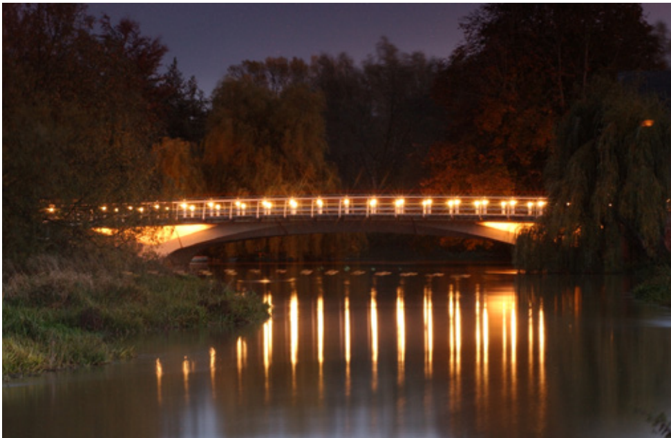
Fig 5.177 Ballingdon Bridge at night, the illuminated bollards light the pavements and road thus avoiding the need for lampposts. The bridge itself is also lit on the upstream side only
