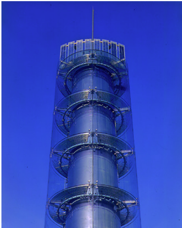
Fig 8.9 The precise curved toughened glass cylinder of the Thames Water Tower crowned by a polycrystalline solar array
