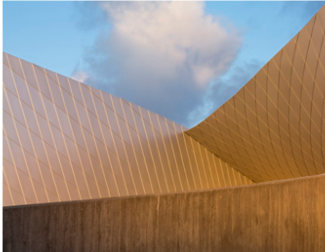
Fig 9.56 Clear PVDF coated aluminium shingles of the Blue Planet reflects the changing environmental conditions of its setting
