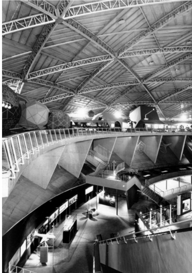
Fig 5.16 The aluminium structure of the Dome of Discovery used repetitive prefabricated elements and had visual clarity
