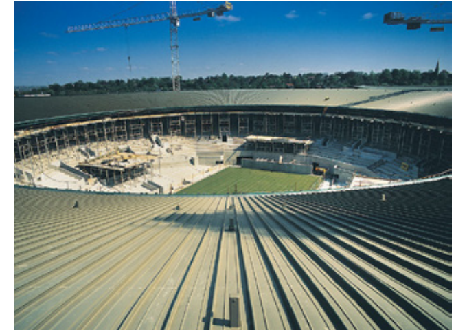
Fig 2.42 The smooth toroidal roof of Wimbledon Number One Court, formed from tapered aluminium standing seam sheeting, architect BDP, 1996
