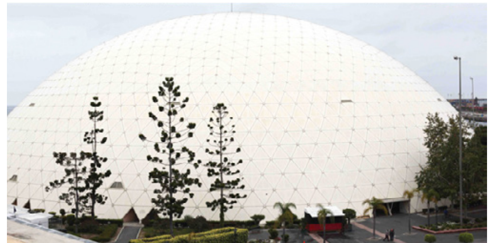
Fig 5.20 The all aluminium, 126m diameter, geodesic Spruce Goose Dome, assembled 1983
