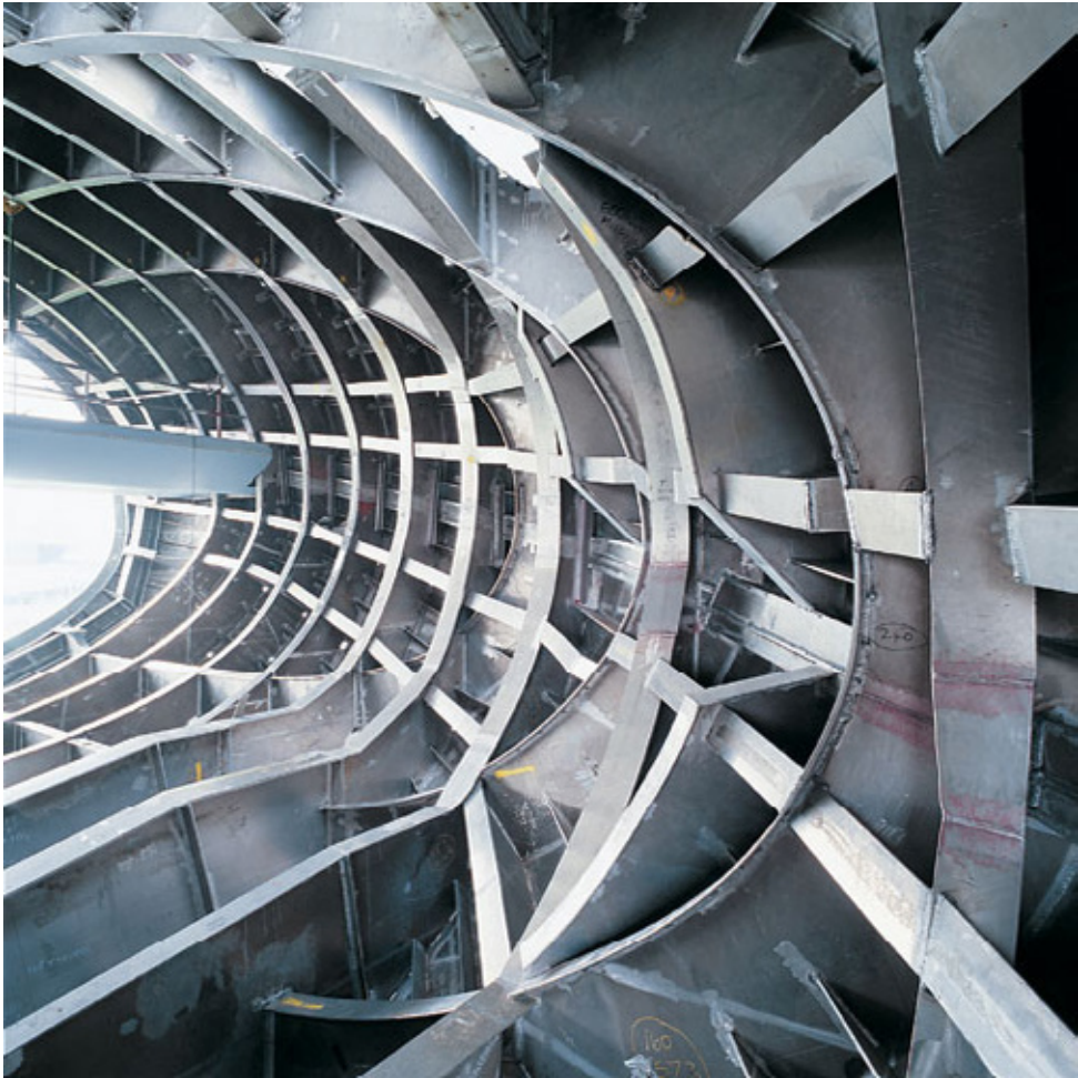
Fig 5.208 The aluminium semi-monocoque structure of Lord's Media Centre
