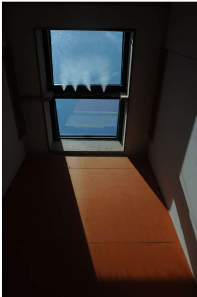
Fig 8.45 PEDC spray system in operation below the rooflights of the Nottingham House
