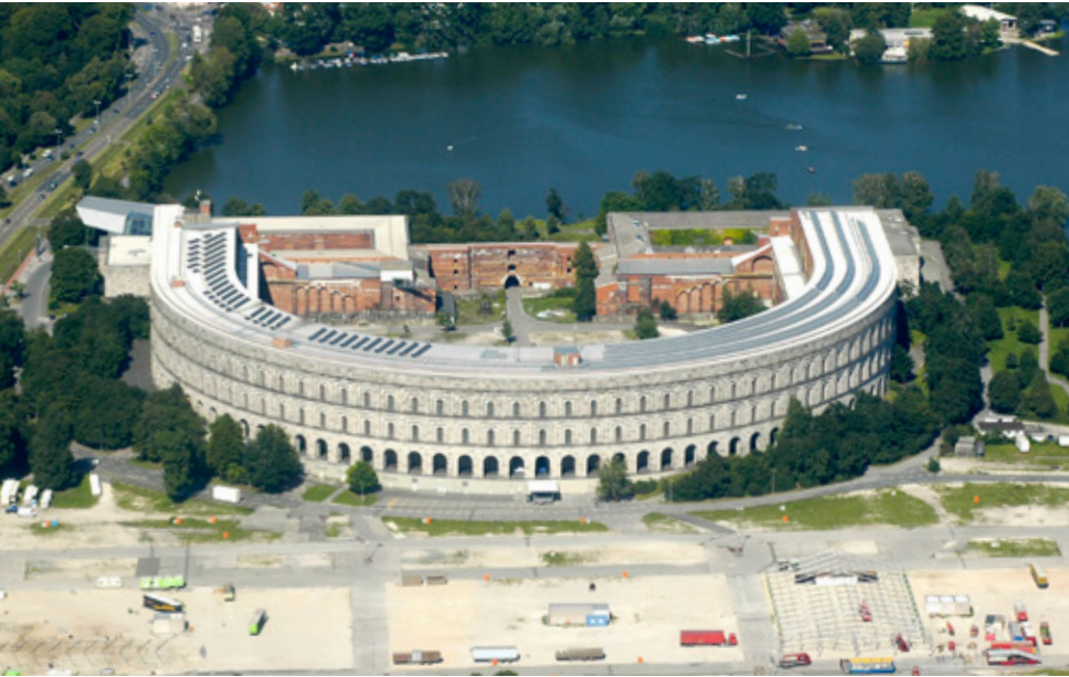
Fig 9.1 Aerial view of Kalzip's profiled aluminium standing seam roof of the Nuremberg Congress Hall, installed in 1968
