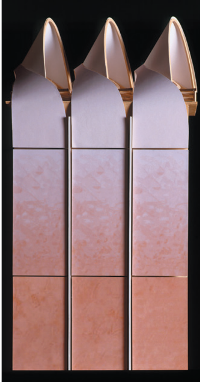
Fig 3.45 At the design stage, represented by this model, the sun cowls and aluminium cladding were separate elements
