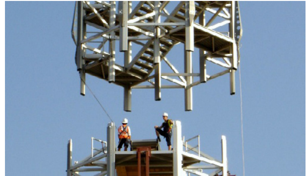
Fig 5.212 The self supporting aluminium stair tower core was prefabricated in large chunks by Bayards
