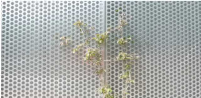
Fig 9.62 The perforated aluminium cladding also provides support for climbing plants
