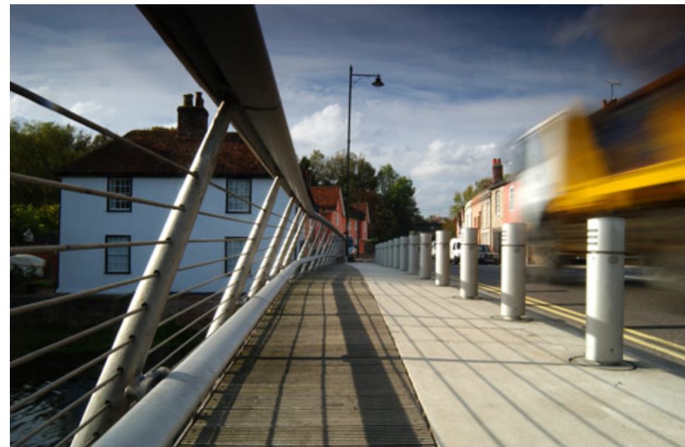
Fig 5.171 The balustrade of Ballingdon Bridge was designed to be visually open yet it is capable of stopping a 42 tonne track form falling into the river Stour
