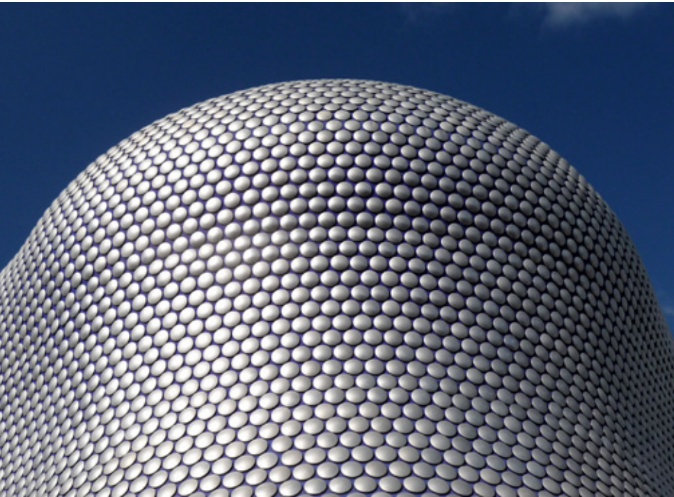
Fig 2.59 15,000 aluminium alloy spinnings form the façade of Selfridges Department Store, photographed 2008
