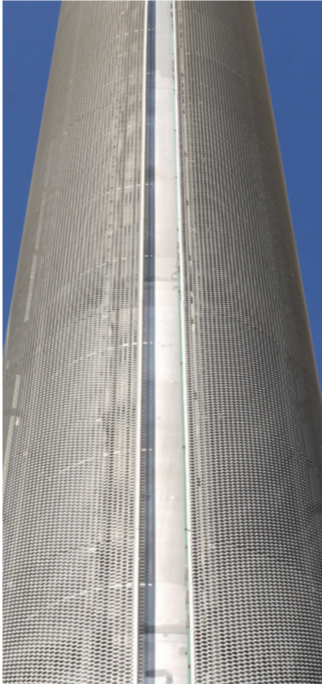
Fig 7.40 The expanded aluminium minimises the vortex shedding and thus limits the possibility of vibration in the i360 tower
