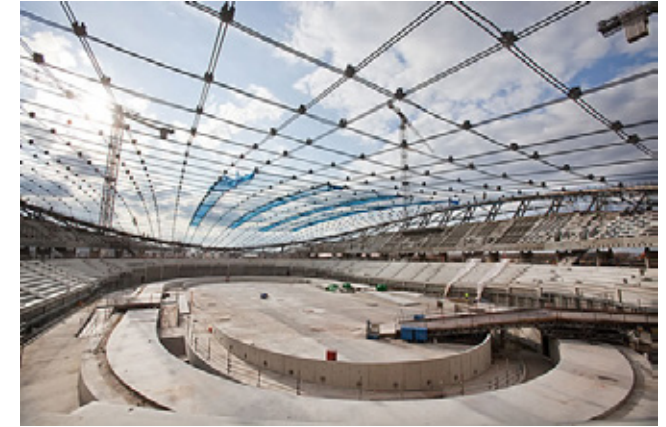
Fig 9.30 The steel cable net tensioned and ready to receive the timber cassette panels
