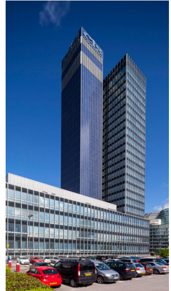
Fig 8.21 CIS Tower, Manchester, England, 1962, overclad with photovoltaic panels in 2005, photographed by Adrian Toon (a2n) in 2016
