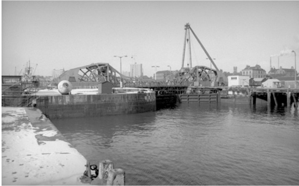
Fig 5.190 St Clements' Aluminium alloy bascule bridge of Victoria Dock in Aberdeen Harbour viewed from Waterloo Quay in 1970
