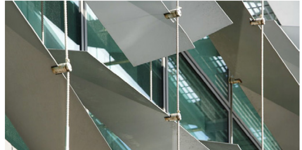
Fig 3.67 Folded and silver polyester powder coated aluminium solar shading of the Children's Eye Centre
