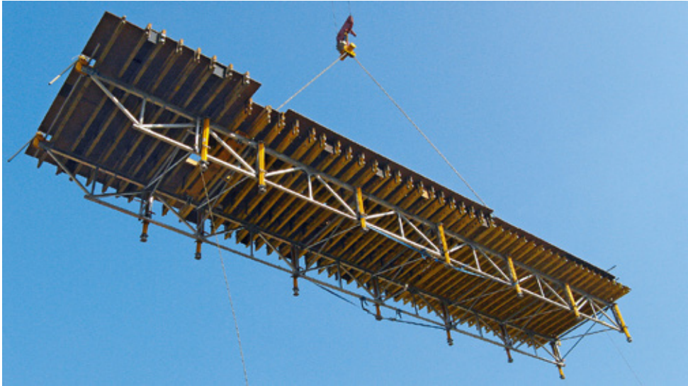
Fig 5.65 100m² PERI SKYTABLE slab formwork being lifted into place at Marina Bay, Singapore, which is made from ply, timber, steel and aluminium
