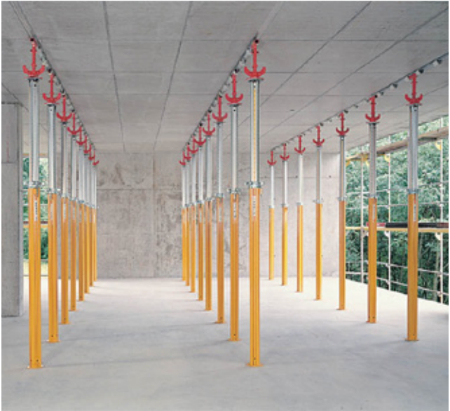
Fig 5.62 Once all the formwork has been struck the MULTIPROPS alone remain in place
