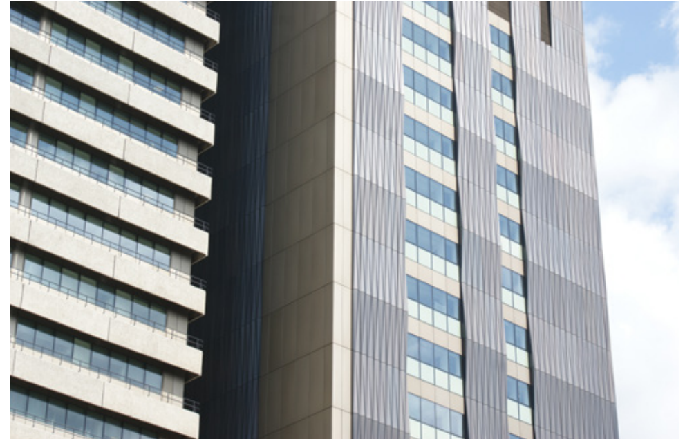
Fig 4.12 The overcladding primarily comprises folded dark grey anodised aluminium rainscreen panels with pale umber anodised aluminium curtain walling and spandrel panels
