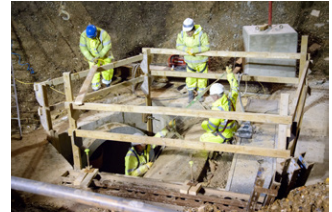
Fig 7.29 Before the foundations of the i360 could be formed, a major sewer had to be diverted
