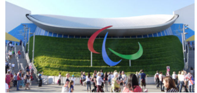
Fig 10.6 London 2012 Aquatic Centre designed by Zaha Hadid Architects for the Olympic Delivery Authority, shortlisted for the Stirling Prize in 2014, its building fabric includes a mill-finish aluminium standing seam roof
