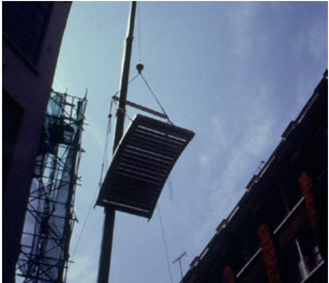
Fig 5.3 Craning the aluminium based prefabricated roof light of the Lowe Apartment, London, designed by Brookes Stacey Randall Fursdon
