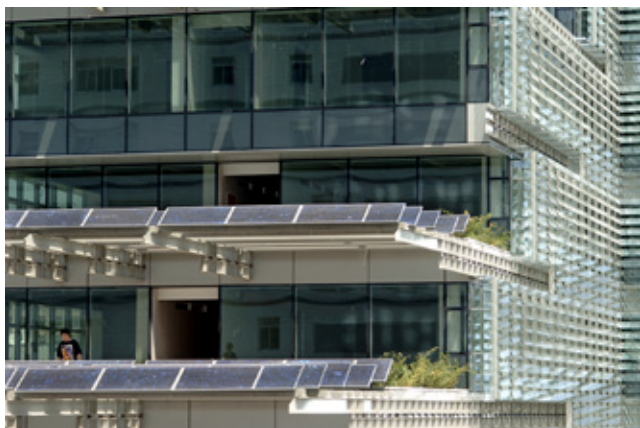
Fig 8.28 The photovoltaic panels also shade the south façades and terraces
