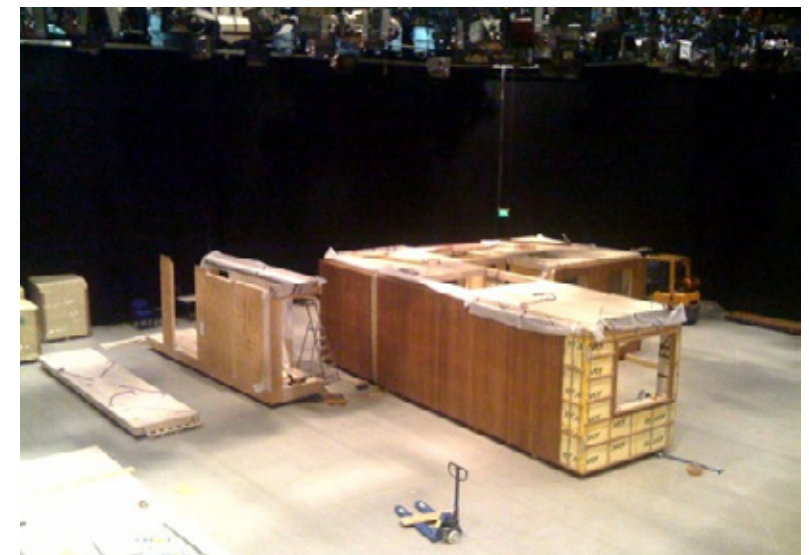
Fig 8.46 Assembling the modules of the Nottingham House in the former Carlton Television Studio
