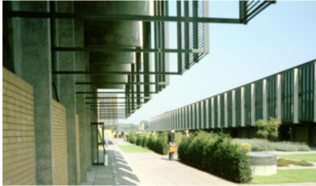
Fig 3.6 Solar shading of St Catherine's College, Oxford, England, architect Arne Jacobsen, completed in 1963
