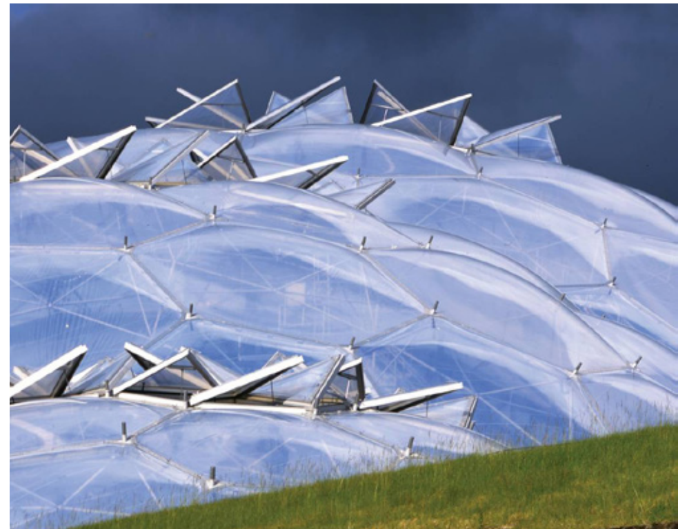
Fig 6.30 Openings in the façade provide ventilation, helping to control the internal environment
