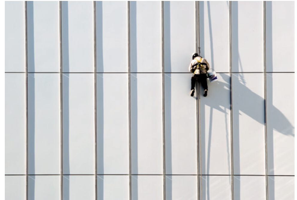
Fig 3.53 An abseiler painting the steel flat between the aluminium rainscreen panels
