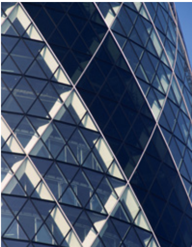
Fig 7.7 The openable double glazing of 30 St Mary Axe, is defined by the dark grey tinted glass, architect Foster + Partners
