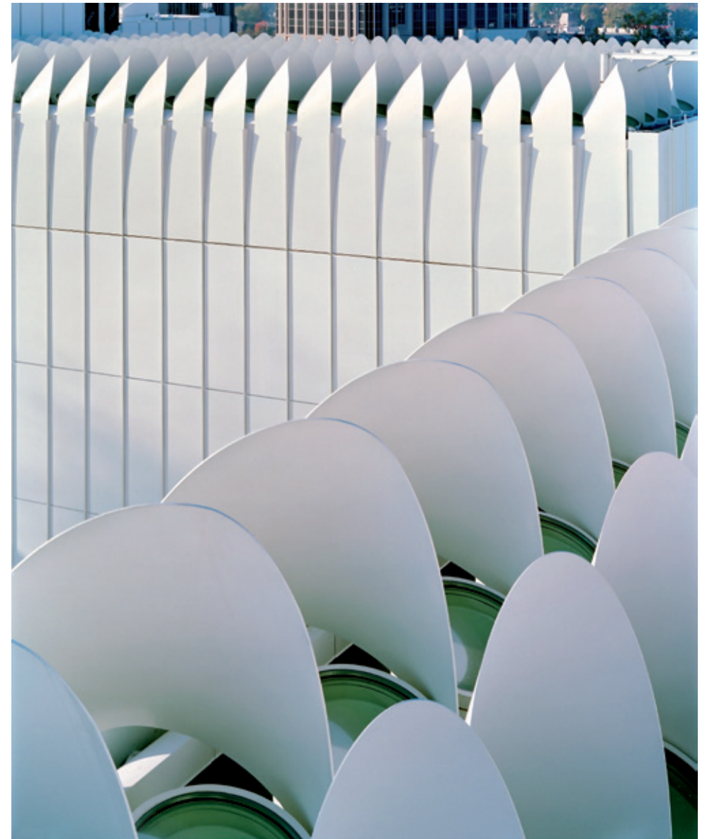
Fig 3.55 Buchanan describes 'the twist to form the cowls along the edge of the roof, one of the most ingenious and beautiful devices ever invented by RPBW
