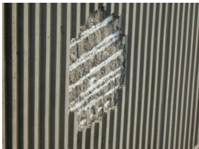
Fig 4.7 When inspected in 1998, the concrete was found to be spalling
