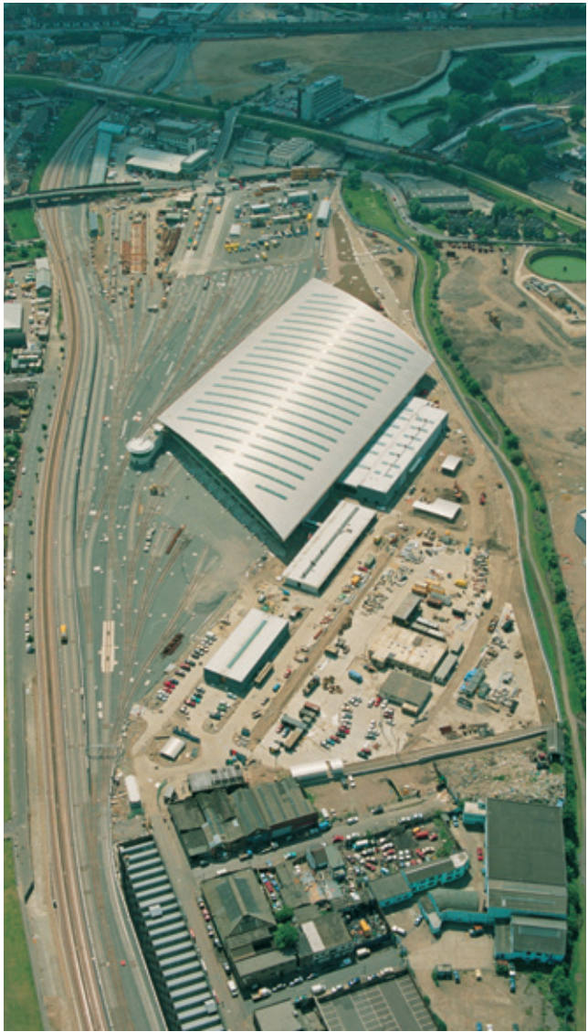
Fig 9.7 The expansive aluminium standing seam roof of Stratford Market Depot
