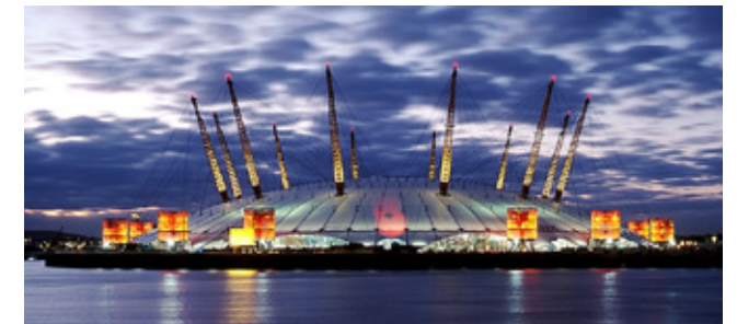
Fig 1.6 The Millennium Dome (O2) designed by Richard Rogers + Partners and completed in 1999 may at first sight only use aluminium louvres to clad the services pods, however the PTFE is secured in maintainable segments by about 24 kilometres of large aluminium extrusions
