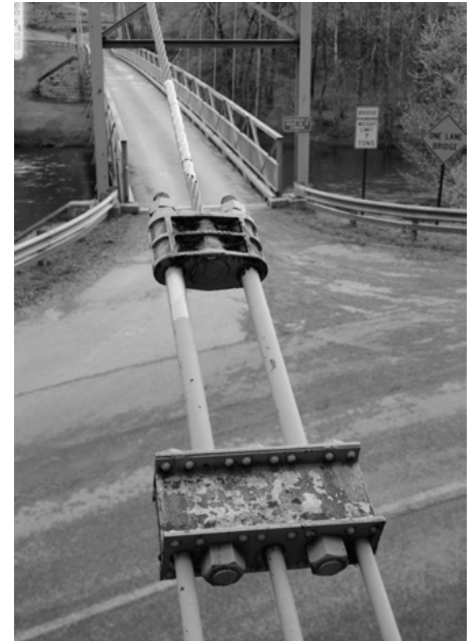
Fig 5.197 Wire rope anchorage detail of Corbin Suspension Bridge
