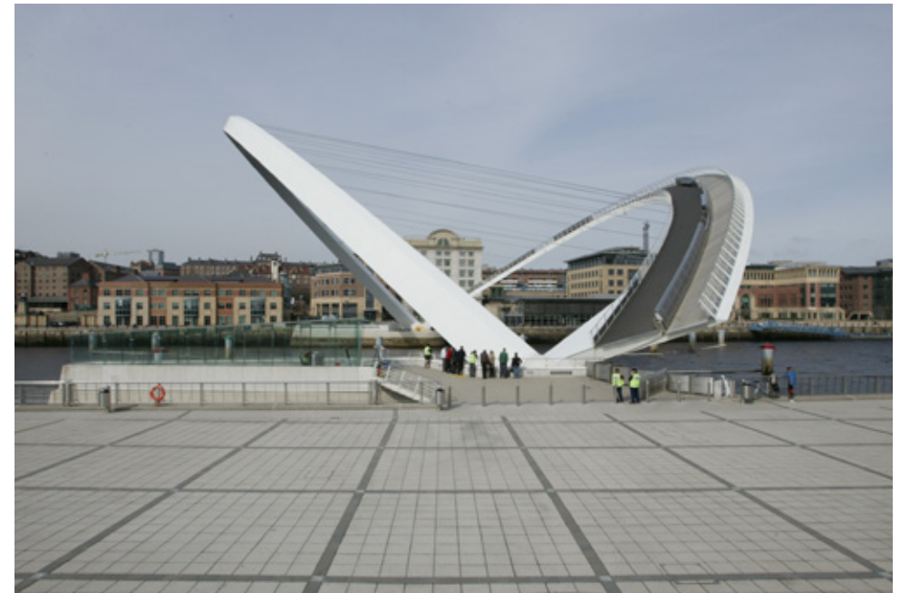
Fig 5.147 The Millennium Bridge, Gateshead, rotated into the open position
