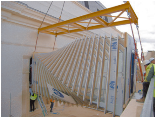
Fig 5.89 Note the precision of prefabricated assemblies as the bridge is eased into place
