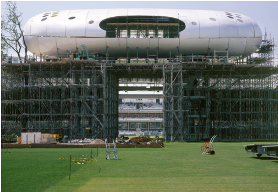
Fig 5.199 Lord's Media Centre under construction clearly showing the prefabricated aluminium components
