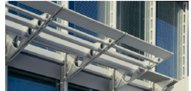
Fig 2.16 Die cast aluminium brise soleil of the Hongkong and Shanghai Bank Headquarters, Foster Associates, 1986
