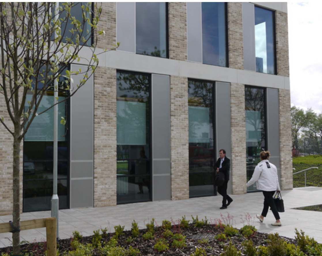
Fig 6.19 The façades of Lancaster University Engineering Building is a careful composition of glazing, perforated anodised aluminium, brick and precast concrete
