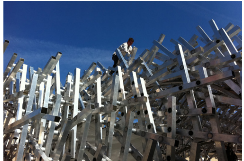
Fig 5.223 The aluminium exoskeleton of the music pavilion being assembled in Salzburg
