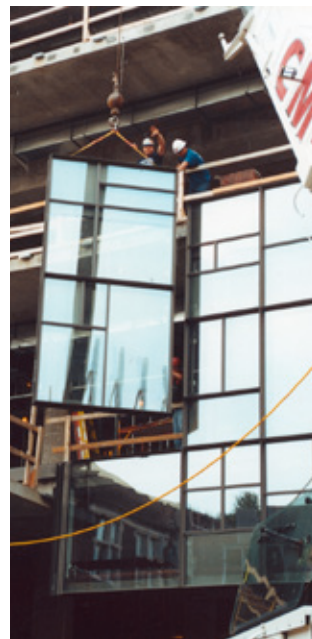
Fig 7.11– Fig 7.13 PermaSteelisa installing the unitised double façade of Melvin J. and Claire Levine Hall
