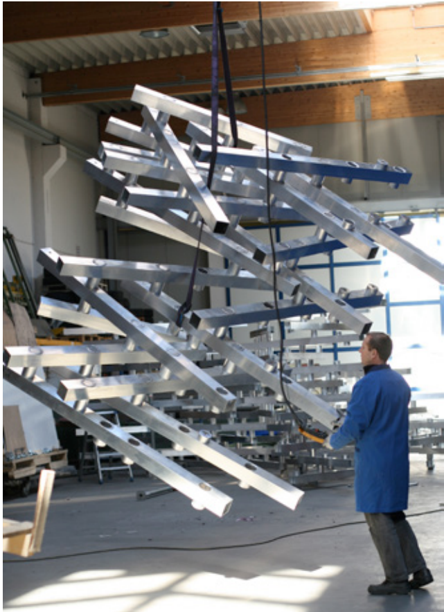
Fig 5.200 The aluminium structure of Vague Formation Mobile Music Pavilion was prefabricated in large but easily craned chunks
