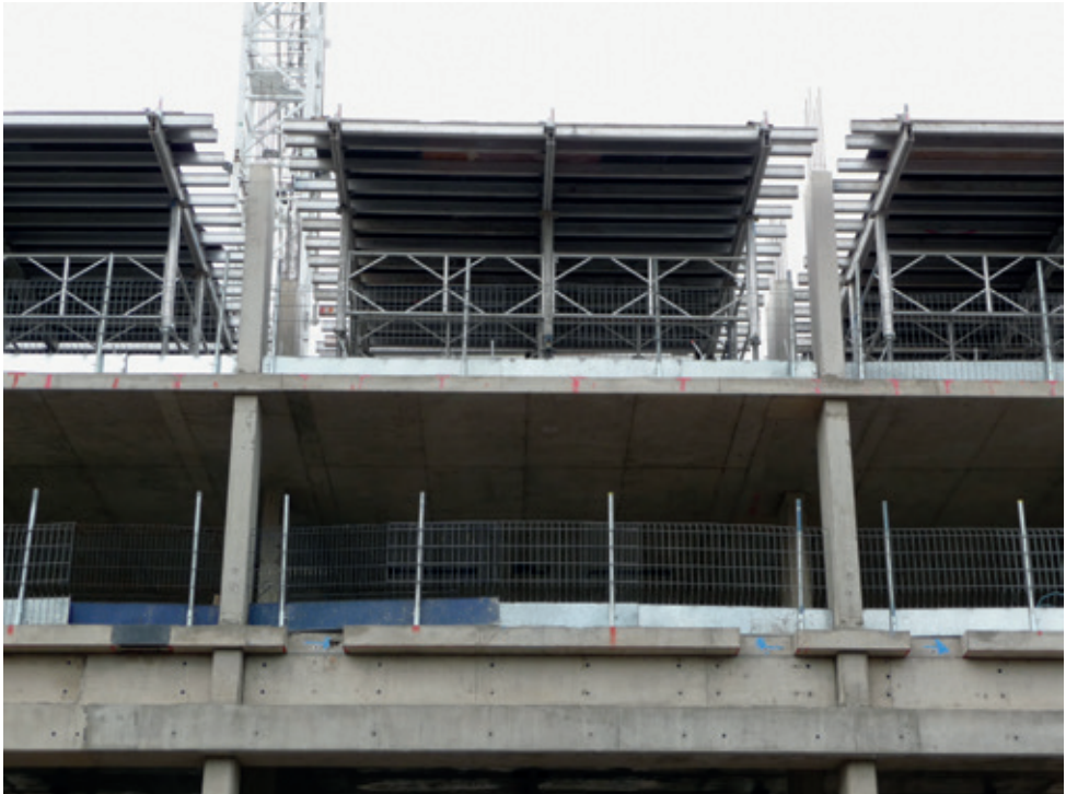
Fig 5.53 Aluminium framed table formwork ready for the casting of the next floor slab, on site at Canal Street, Nottingham
