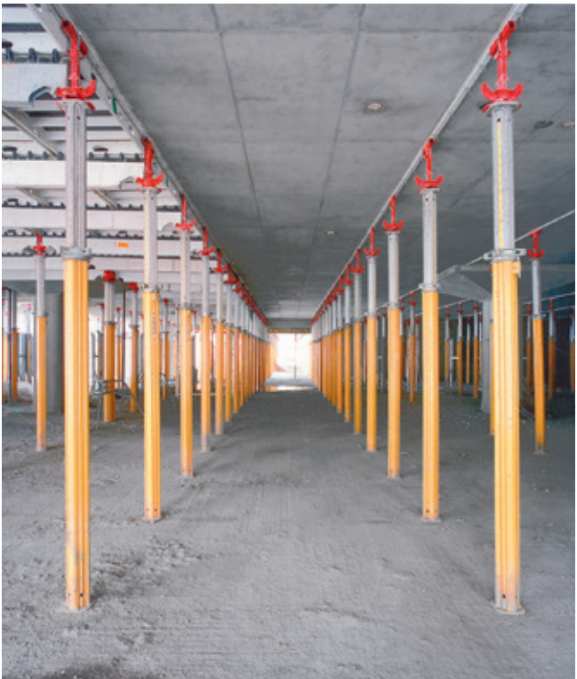
Fig 5.61 The dropheads enables the early striking of the formwork
