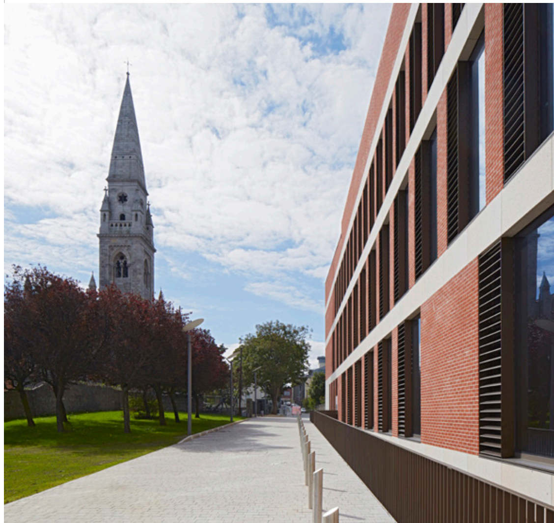
Fig 6.54 Haigh Terrace elevation, bronze anodised aluminium louvres and window set in a façade of brick and stone
