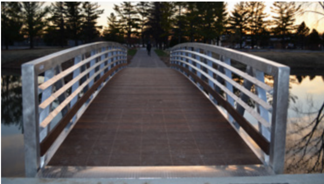
Fig 5.97 Equestrian Park Bridge, an aluminium bridge with a hardwood deck, designed and fabricated by MAADI Group
