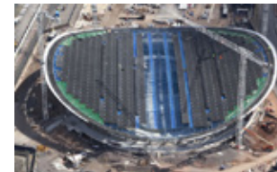
Fig 9.31 Installing the timber cassette panels on the tensioned steel cable net
