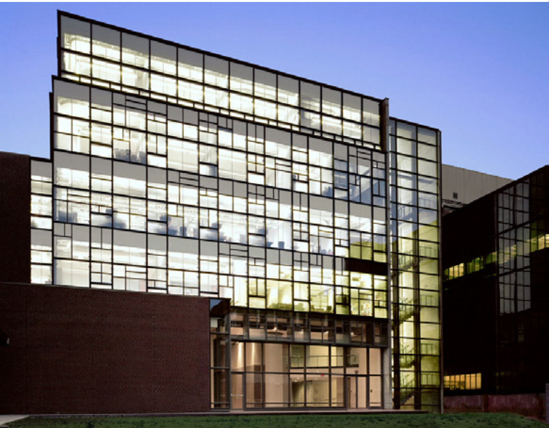
Fig 7.9 Melvin J. and Claire Levine Hall, designed by KieranTimberlake, the first use of an active double façade in the USA
