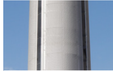
Fig 7.41 Gaps for the four masts of the pod where it climbs the tower delineate the anodised expanded aluminium cladding and further emphasising the slenderness of the tower
