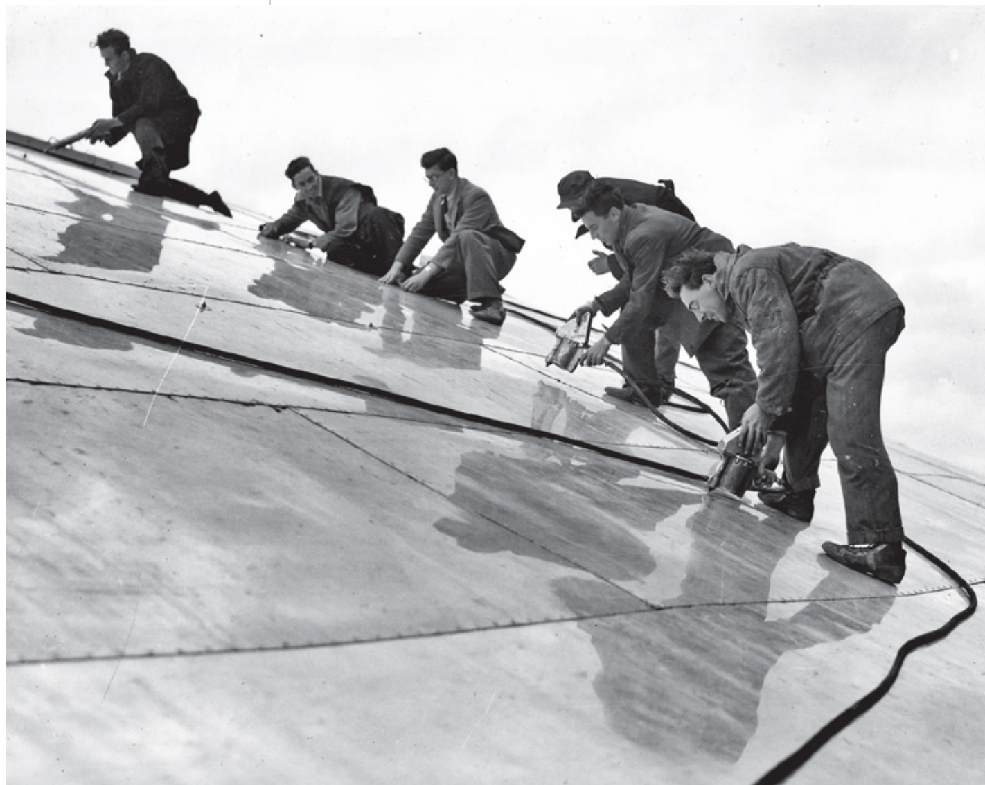
Fig 9.4 Riveting the aluminium cladding of the Dome of Discovery at the Festival of Britain, architect Ralph Tubbs, 1951
