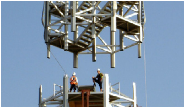
Fig 5.201 The self supporting aluminium stair tower core was prefabricated in large chunks by Bayards
