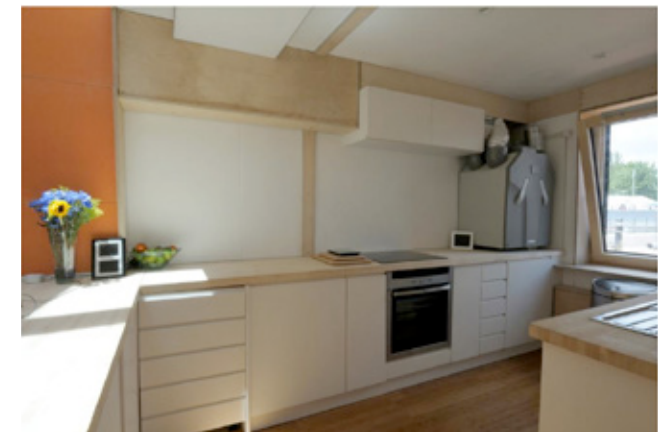
Fig 8.43 The whole house heat recovery system is left exposed in the kitchen
