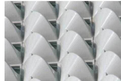
Fig 2.17 Cast aluminium shells of the solar shading at the Nasher Sculpture Center, designed by Renzo Piano Building Workshop, 2003
