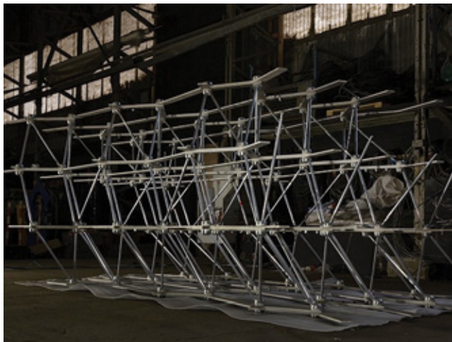
Fig 2.139 Trial assembly of a layer of the meshwork structure of the Hive
