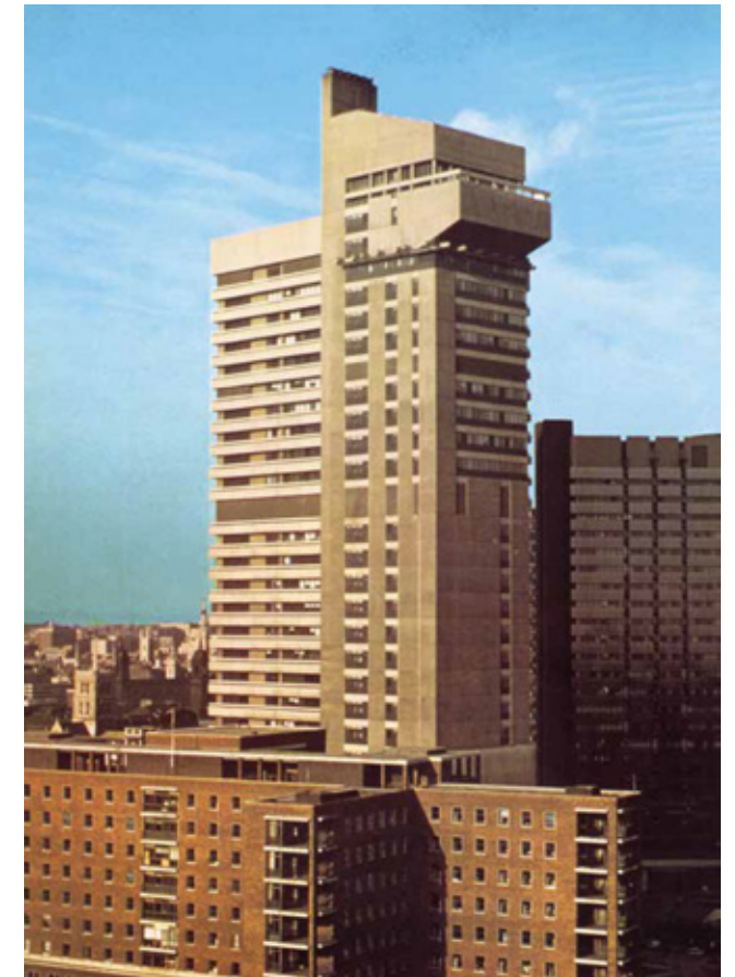
Fig 4.6 Guy's Hospital Tower designed by Watkins Gray Architects and completed in 1974, note the vertically ribbed concrete of The Communications Tower and the whiter horizontal balconies of the User Tower
