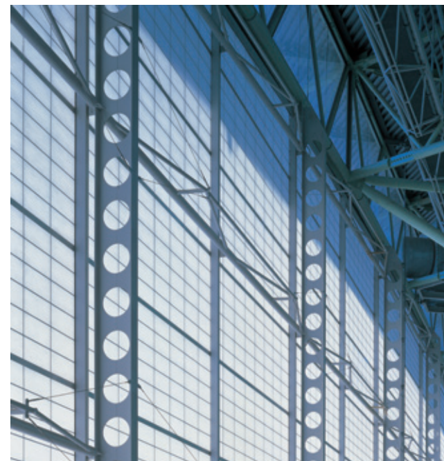
Fig 9.10 The south west façade of the Depot is clad with Kalwall
