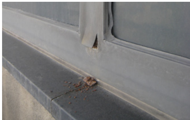
Fig 4.8 The inspection also found the steel windows were corroding badly
