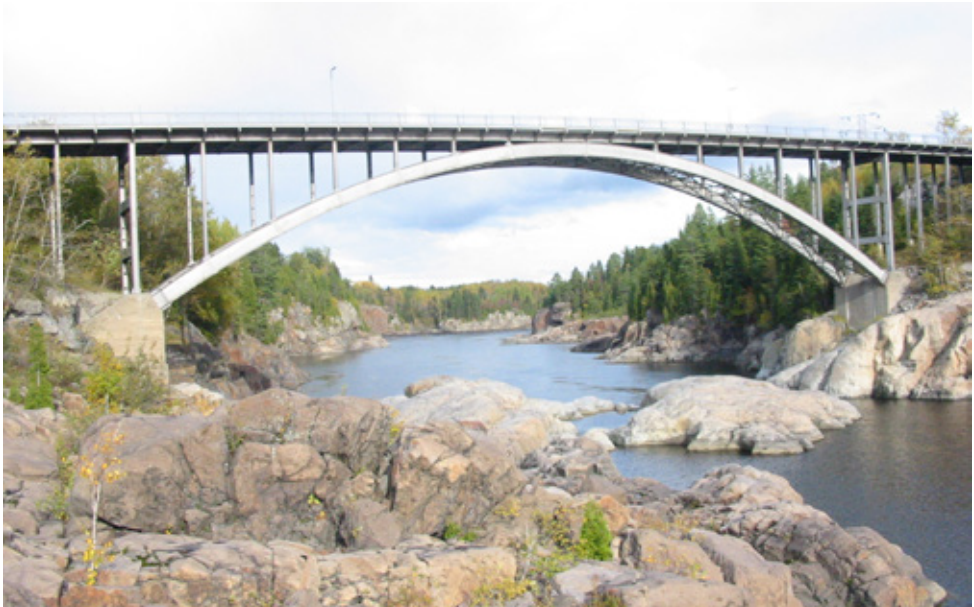
Fig 5.193 Arvida Bridge an all aluminium road bridge spanning the Saguenay River, 1950
