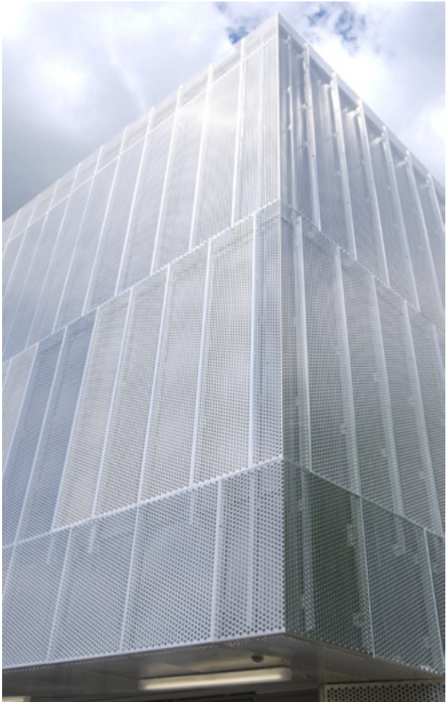
Fig 9.61 The perforated aluminium sheet is simply folded to form the corner of the east and south façades
