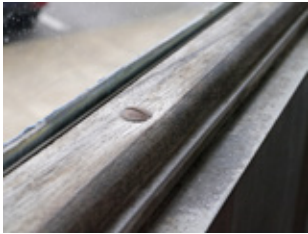
Fig 5.23 Screw fixed and unpainted hardwood glazing bead of a vision panel, photographed 2016
