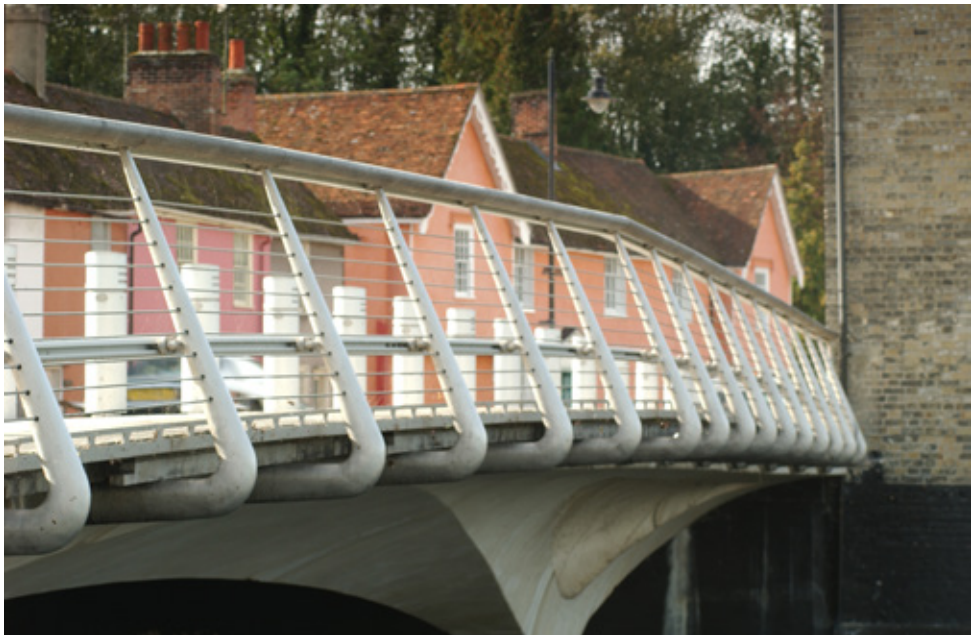
Fig 5.175 Visually open balustrade of Ballingdon Bridge
