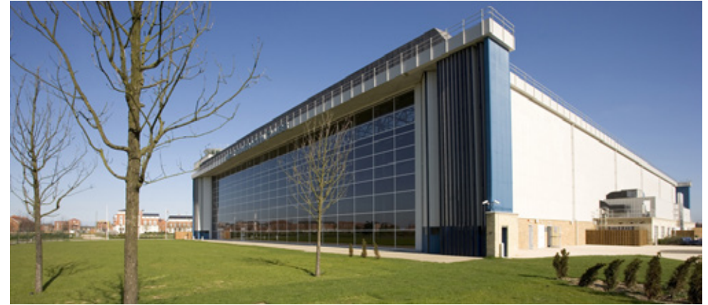
Fig 5.32 After conversion the doors of the south elevation are fixed open and a double glazed curtain walling has been installed
