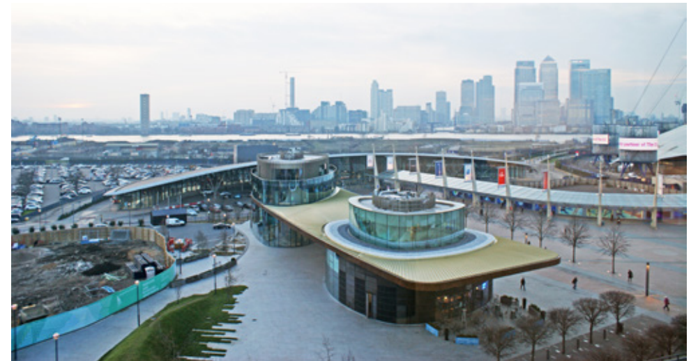
Fig 2.43 Greenwich Gateway Pavilions, Marks Barfield Architects, 2014, gold finished aluminium standing system roof installed by Lakemere, using both tapered and Kalzip XT sheets, delivered by the collaborative use of a Building information model (BIM). The gold finish is produced by an electrolytic passivation process
