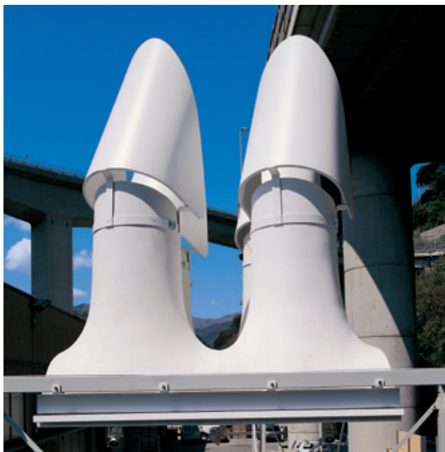
Fig 3.39 Prototypes of the aluminium sun cowls or velas
