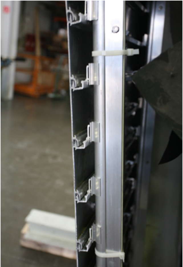
Fig 4.36 Detail of the gasketed extruded aluminium cladding and carrier system
