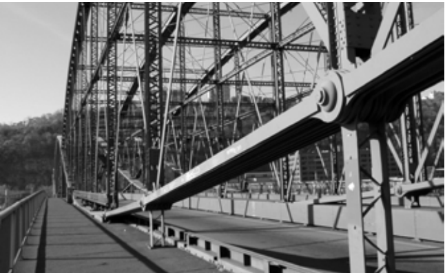
Fig 5.187 Smithfield Street Bridge, Pittsburgh, completed in 1882 decking replaced with aluminium in 1933
