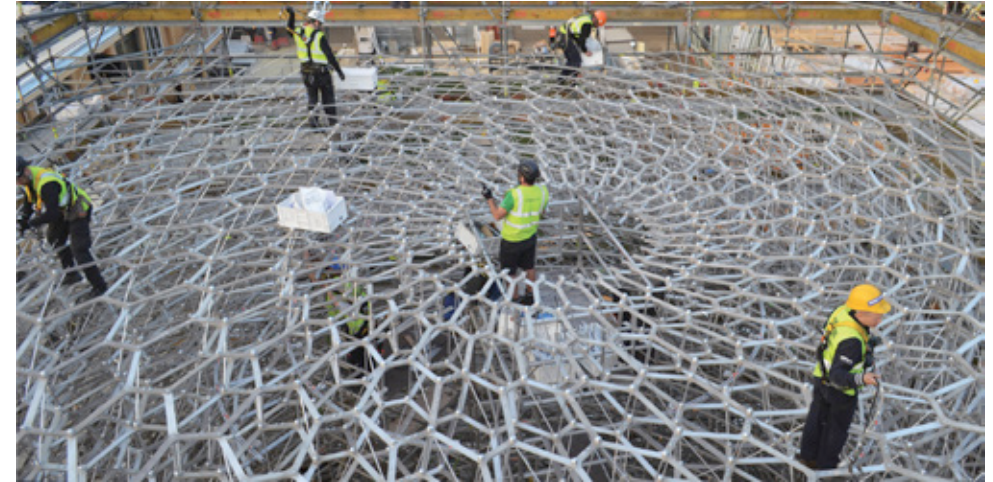
Fig 2.145 The aluminium meshwork structure of the Hive being assembled by Stage One in Milan
