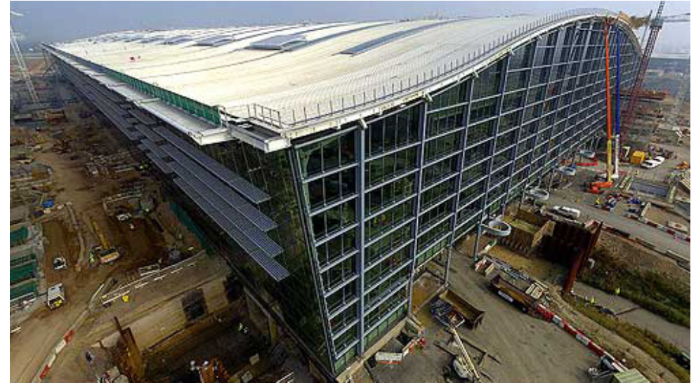
Fig 2.33 The continuous single sheet aluminium standing seam roof of Heathrow Terminal Five, architect Rogers Stirk Harbour + Partners, 1988–2008
