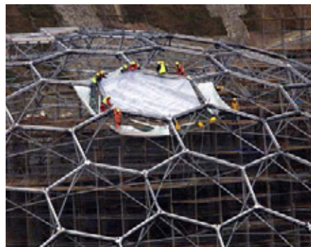
Fig 6.34 The first ETFE pillow being installed on the aluminium hexagonal grid
