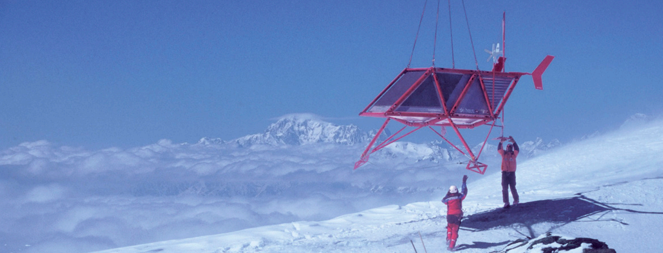
Fig 5.7 The Ski Haus designed by Richard Horden Architects being lowered into place in the Alps
