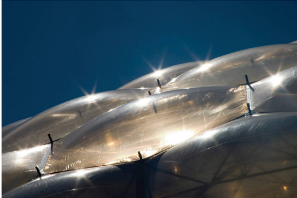
Fig 6.32 The nodes provide articulation to the building fabric with the ETFE providing light in during the day and views of the sky at night
