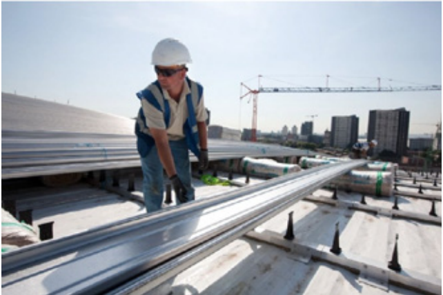
Fig 9.39 Installing the aluminium standing seam roof sheets onto the thermally efficient fixing clips
