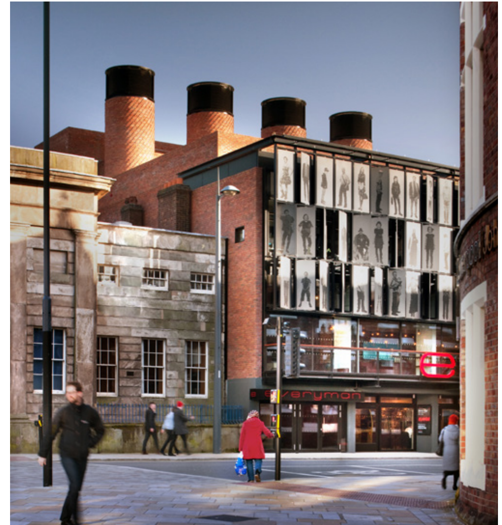
Fig 10.7 Everyman Theatre, designed by Haworth Tompkins for Liverpool and Merseyside Theatres Trust, winner of the Stirling Prize in 2014, its building fabric includes black anodised waterjet cut solar shading
