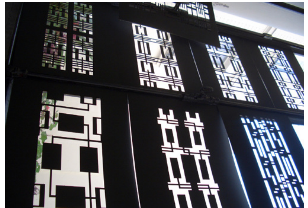
Fig 2.96 Options for the perforated aluminium solar screens
