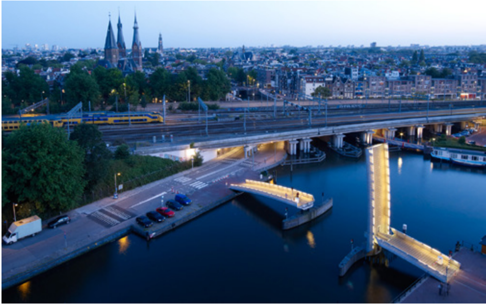
Fig 5.94 Westdork Bridge reveals that it is a 16m leaf bascule
