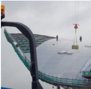
Fig 9.37 Installation of the standing seam aluminium roof of the Aquatics Centre
