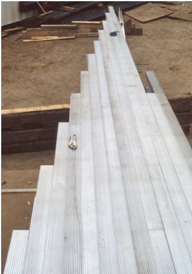
Fig 5.123 The curved plan is achieved by slipping and gently curving the aluminium extrusion in a process of gradual lamination
