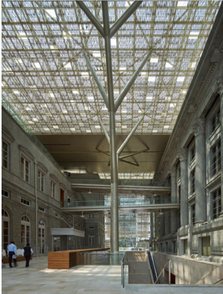
Fig 3.11 The filigree aluminium solar shading in a range of silvers and shades of gold of the National Gallery, Singapore designed by architect studioMilou, which opened during November 2015, was sourced from Guangzhou in China by Beijing Jangho Curtain Wall Co
