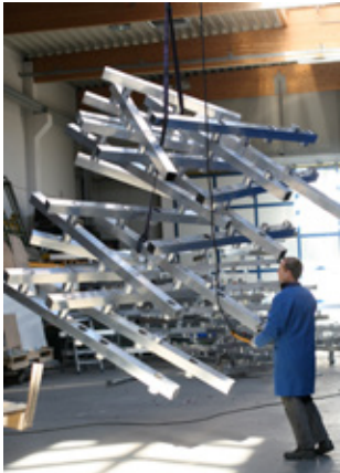
Fig 5.219 The aluminium structure was prefabricated in large but easily craned chunks
