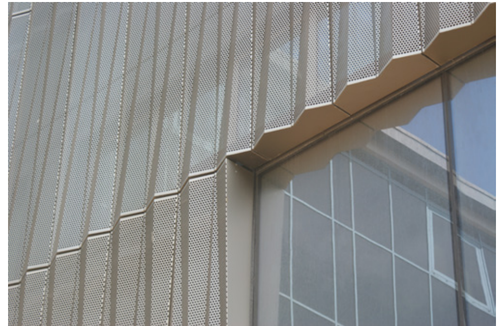
Fig 4.20 [below] Junctions between the folded aluminium cladding and the glazing are carefully considered
