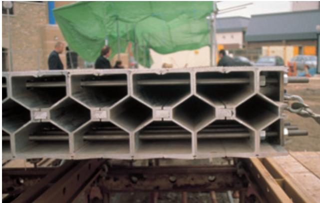
Fig 5.122 Stiff structural cells are formed by post tensioning – achieving a slender deck
