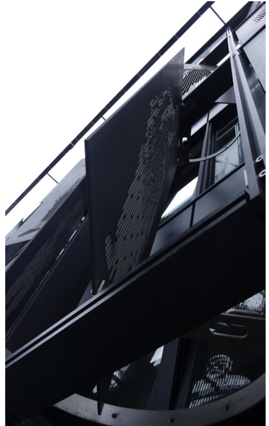
Fig 2.112 8mm thick waterjet cut anodised aluminium solar shading of the Everyman Theatre, Liverpool, England, architect Haworth Tompkins
