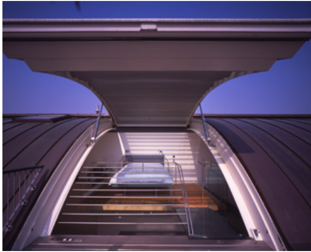
Fig 5.4 The rooflight forms a complete section of roof the Lowe Apartment, architect Brookes Stacey Randall Fursdon, which opens up to enable the owner to sleep under the stars, even in central London
