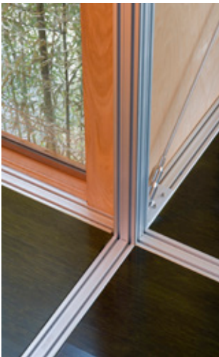
Fig 2.6 Exposed structural aluminium framing and interior detailing at Loblolly House, a private residence in Maryland, USA, designed by KieranTimberlake
