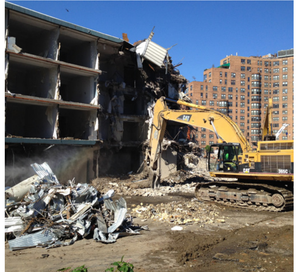
Fig 4.11 Demolition and material sorting. Philadelphia, PA, USA
