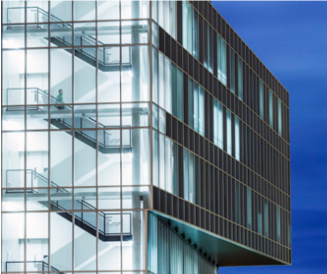
Fig 2.2 Aluminium and glass curtainwall compose the three principal faces of this tower, at Center City Building, University of North Carolina at Charlotte, USA, designed by KieranTimberlake. A pattern of transparent, fritted, and opaque panels screen solar radiation while maximizing natural light and views and working seamlessly with a concrete and steel structure
