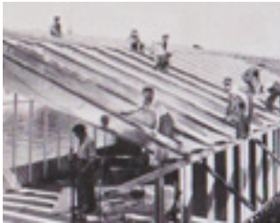
Fig 4.30 Construction of the pavilion in Paris
