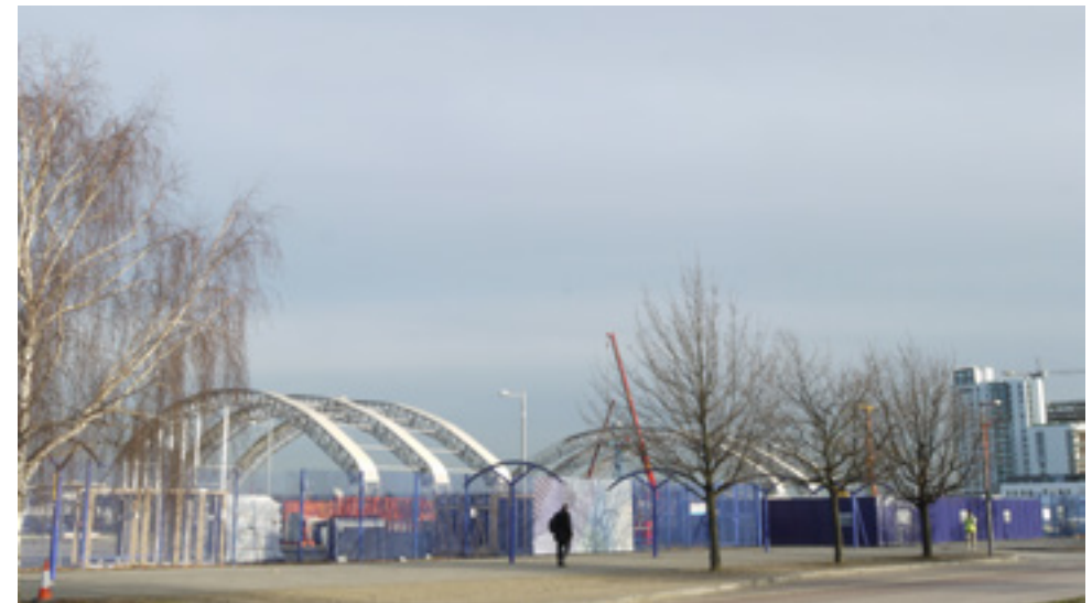
Fig 3.51 The Football Soccer Dome being disassembled, early 2015
