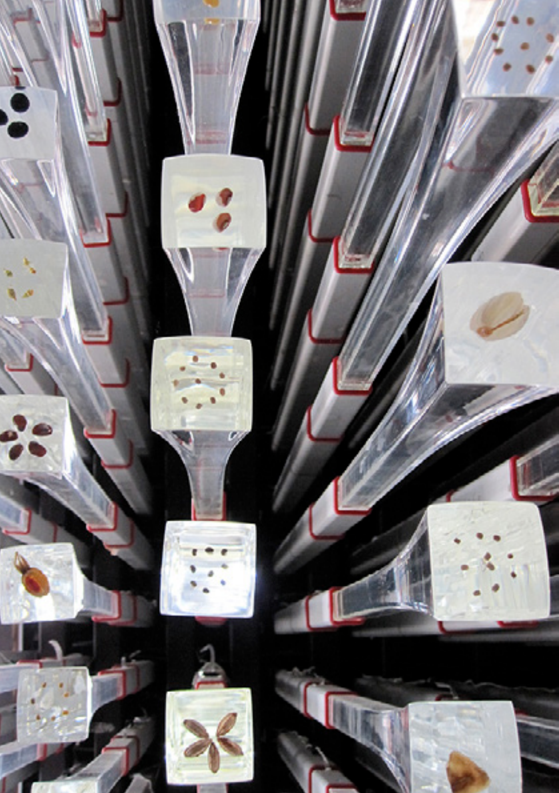
Fig 4.85 [left] Acrylic rods with seeds cast in the tip, showing aluminium sleeve and red plastic extrusions
