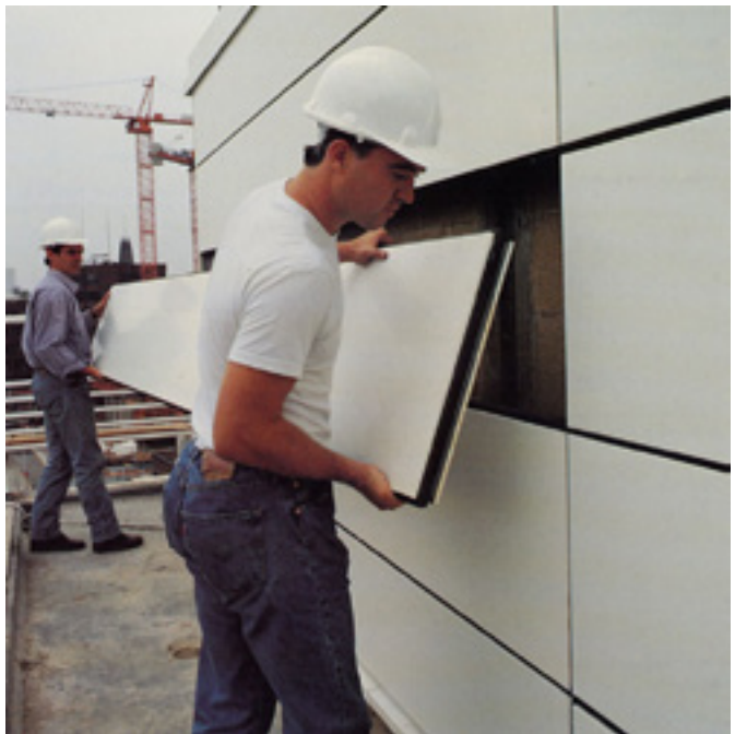
Fig. 2.47 Aspect 2 cladding system installation
