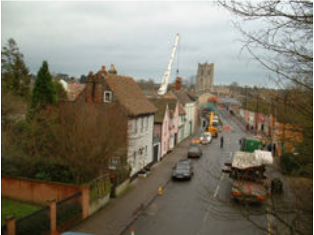
Fig. 2.11 Reconstruction of Ballingdon Bridge on a tight urban site – the temporary Bailey Bridge being lifted into place
