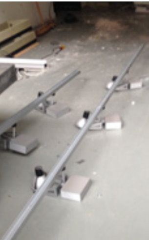
Fig. 5.2 [below] Extruded aluminium lighting support track with lights in situ being stripped from a shop interior, Nottingham, 2015 – these components could be reused or recycled
