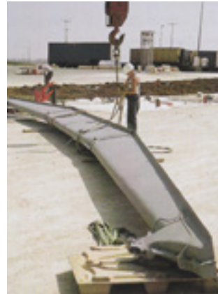
Fig 4.47– Fig 4.51 The beams being restored, ready for reassembly in Villepinte
