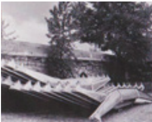
Fig 4.28 Assembled beams on site in Paris
