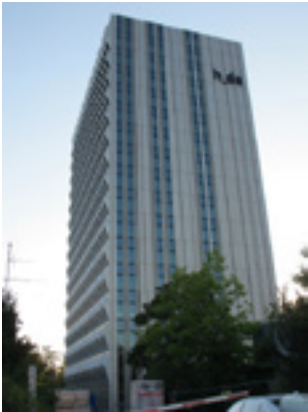
Fig 2.73 The C10 Tower with a new skin of aluminium curtain walling
