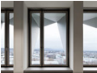
Fig 2.72 Inside the C10 tower, the folded aluminium façade components provide solar shading
