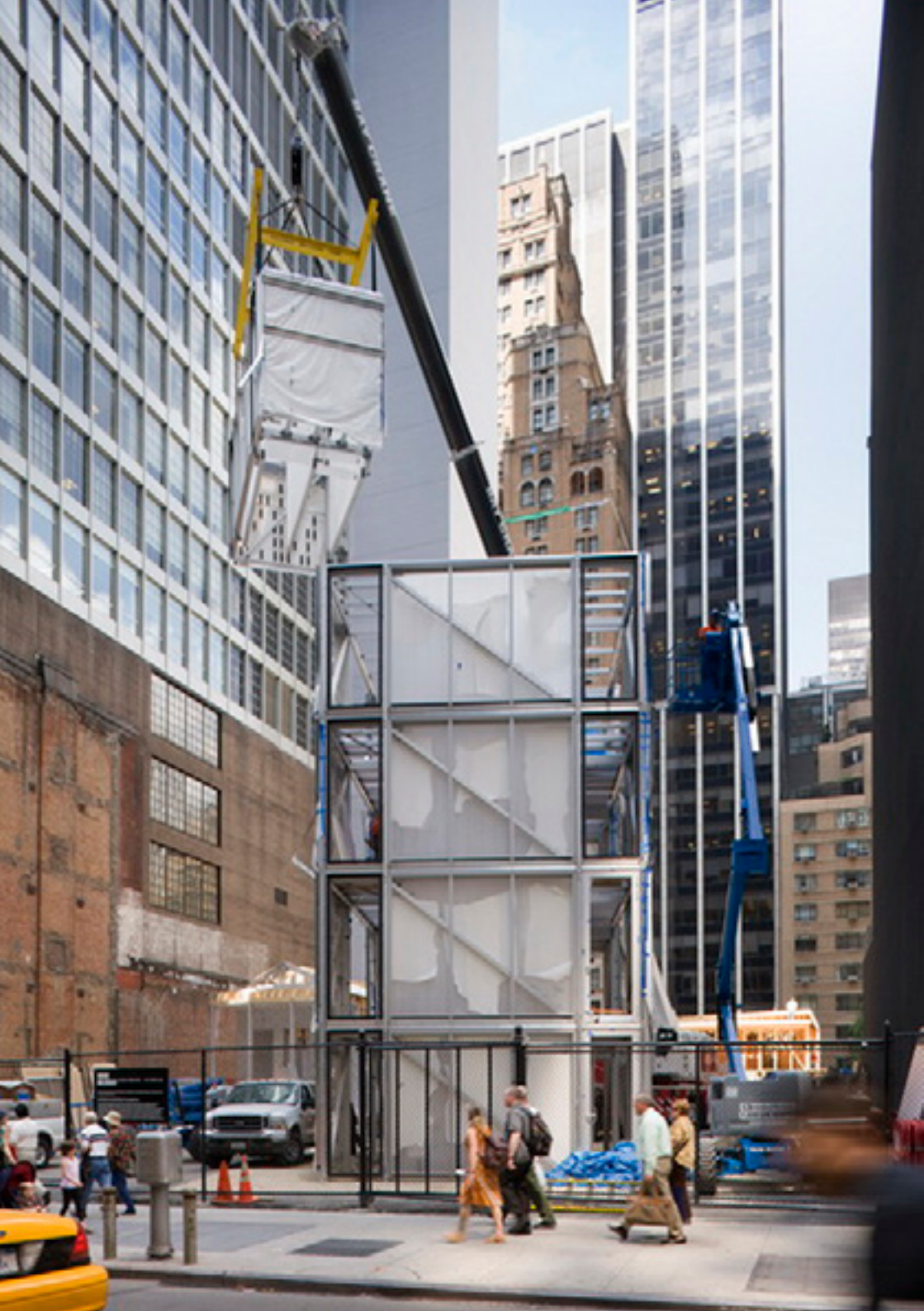
Fig 4.67 [left] Cellophane House™ being assembled in prefabricated chunks
