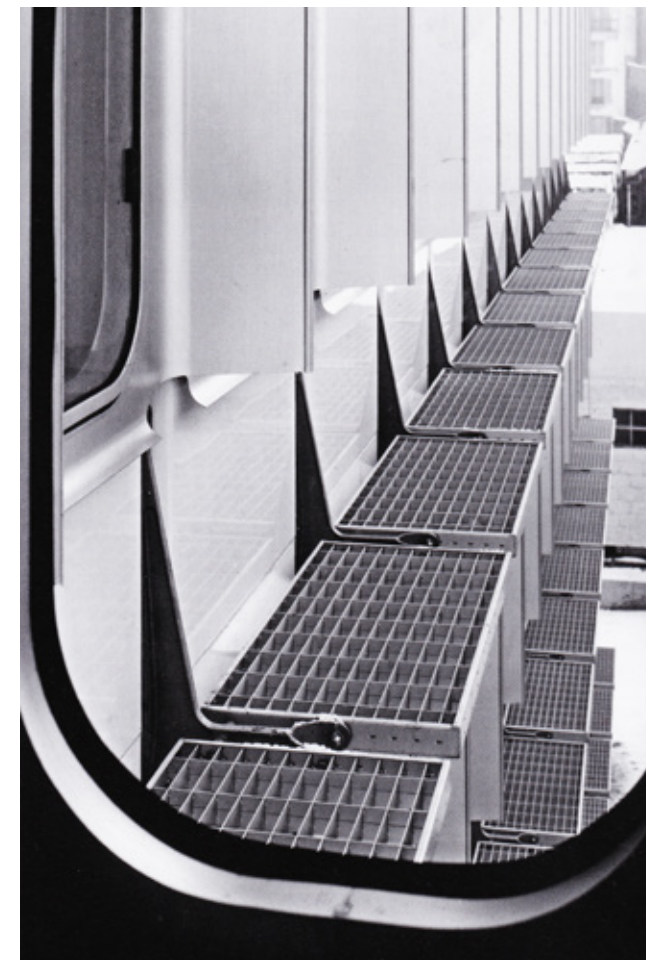
Fig 3.91 Curved, anodised aluminium sheets of the façade of UNESCO Building 5, Paris form integrated solar shading
