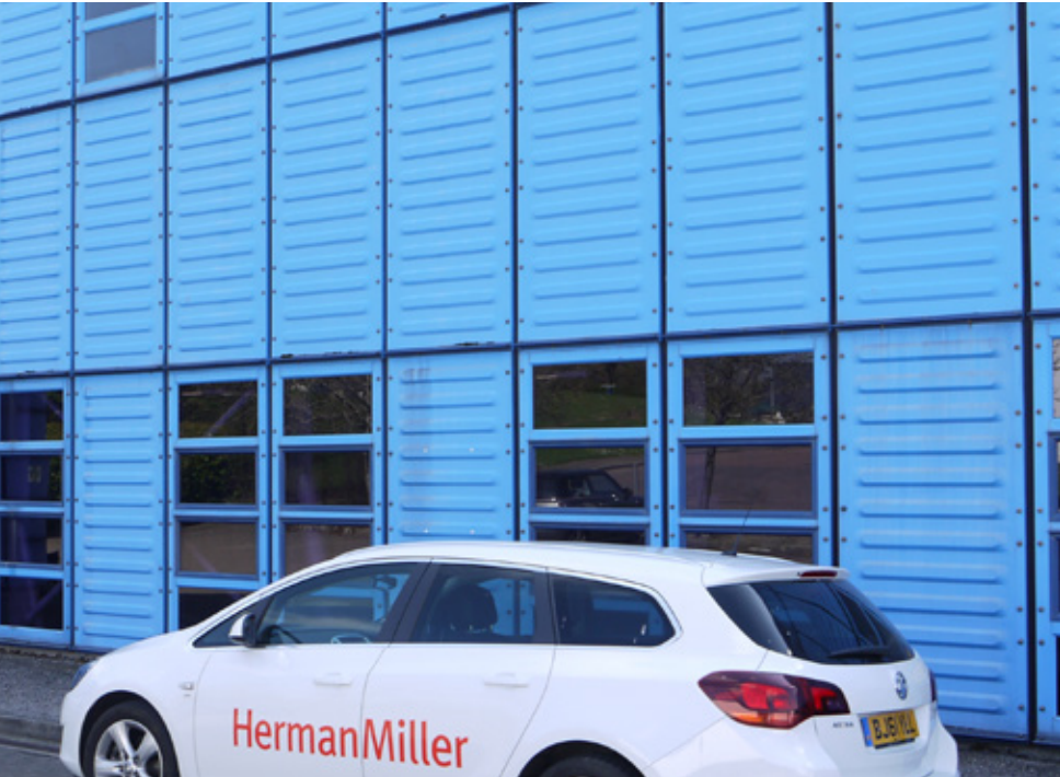
Fig 5.19 Herman Miller Distribution Centre, Chippenham: light blue polyester powder-coated pressed aluminium cladding
