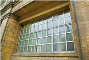
Fig 3.20 Anodised aluminium window of the New Bodleian Library, Oxford
