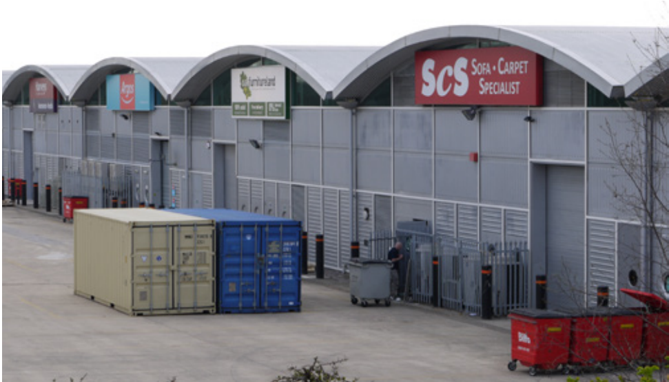
Fig 5.59 Rear loading bay façade: polyester powder-coated pressed aluminium
