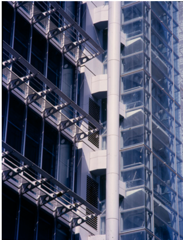
Fig 3.107 Die cast aluminium brise soleil, curtain walling and cladding of the Hongkong and Shanghai Bank Headquarters
