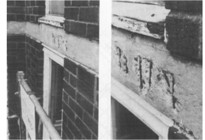
Fig 5.52 Parsons House prior to over-cladding: spalling concrete and rotten timber windows
