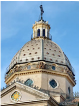
Fig. 7.2 The mill-finish aluminium cladding of the dome of San Gioacchino, Rome, 1897, architect Raffaele Ingami
