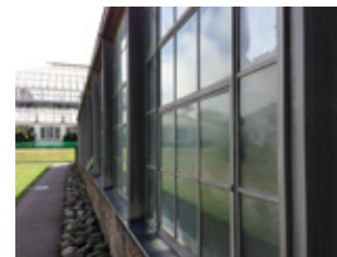
Fig 3.39 Detail of the aluminium façade of Evolution House, Kew Gardens
