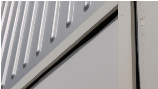
Fig 5.69 Peeling over-painted polyester powder coating found at Cribbs Causeway Building A
