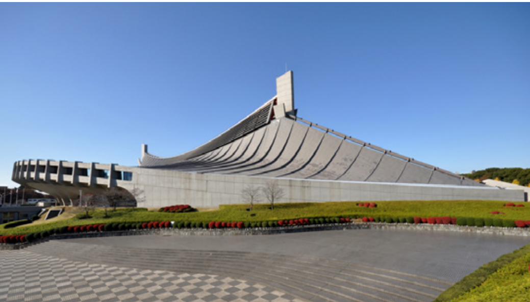
Fig 3.86 Suspended aluminium roof of the National Olympic Gymnasium, Tokyo
