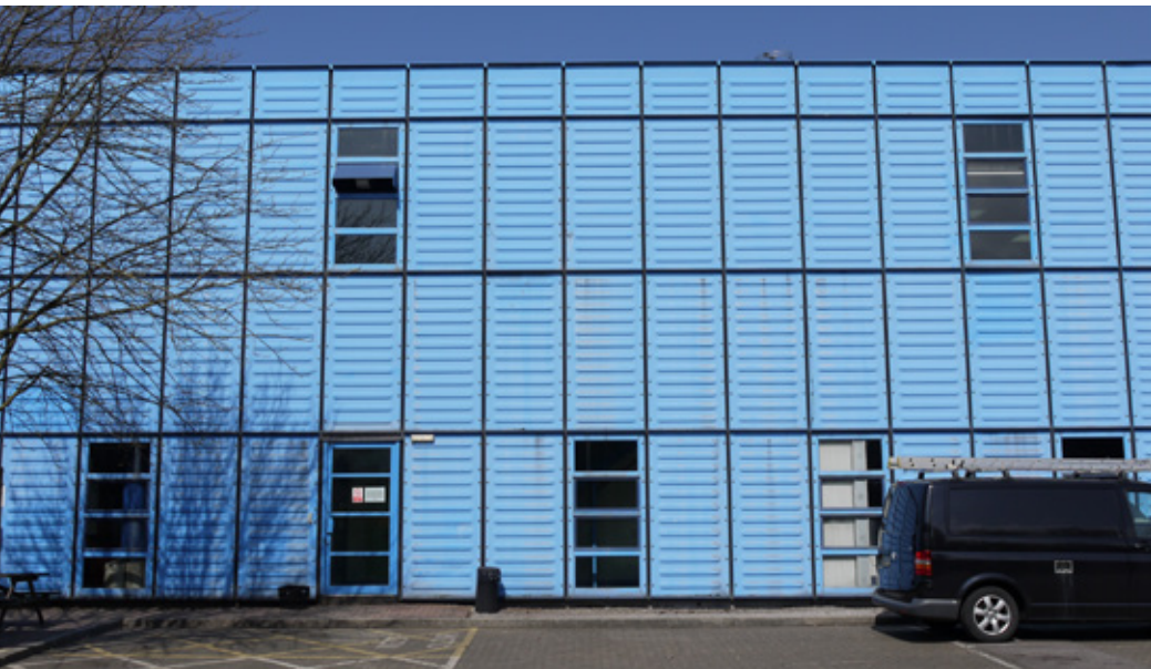
Fig 5.31 Polyester powder-coated pressed aluminium interchangeable panels and windows of the south façade
