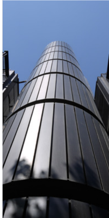
Fig 5.37 Bronze anodised extruded aluminium cladding on the stair tower of 1 Finsbury Avenue, architect Arup Associates, 1985
