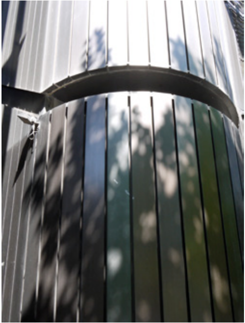
Fig 5.41 [below] Expressed cruciform of the bronze anodised curtain walling
