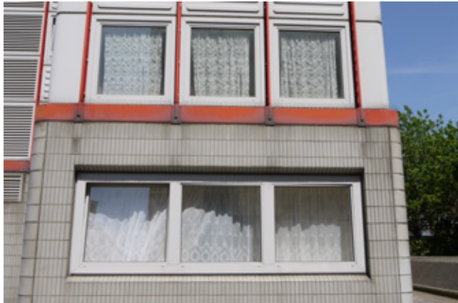
Fig 5.54 Tiled base of Parsons House: note the anti-pigeon measures and the staining to the tiles
