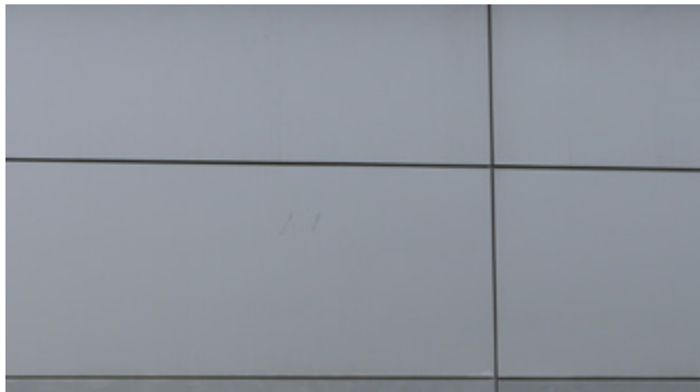
Fig 5.67 Cribbs Causeway Building B Front elevation: polyester powder-coated pressed aluminium panels in a curtain-wall system
