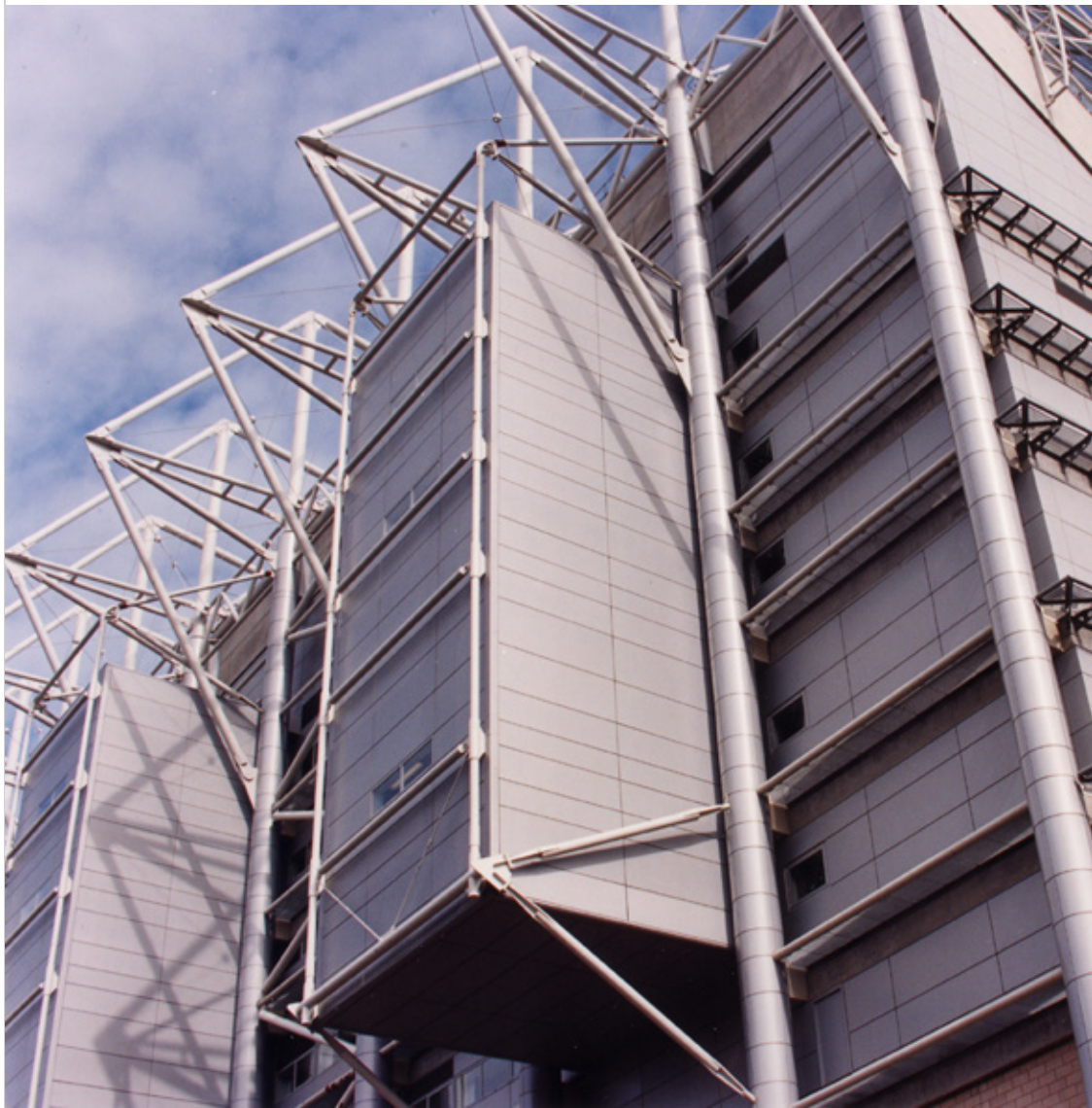
Fig 5.70 St James' Park, Newcastle, clad in Aspect 3, integrated composite metal panel system – invented, designed, developed and tested by Michael Stacey
