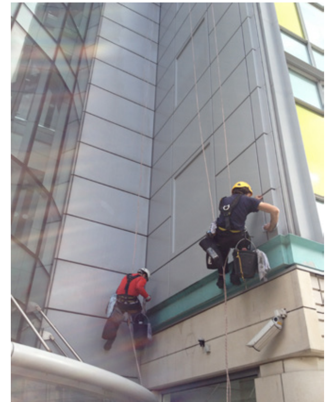
Fig 7.6 Holiday Inn Express, Nottingham: abseilers cleaning the aluminium cladding, 13.53pm on 6 October 2012
