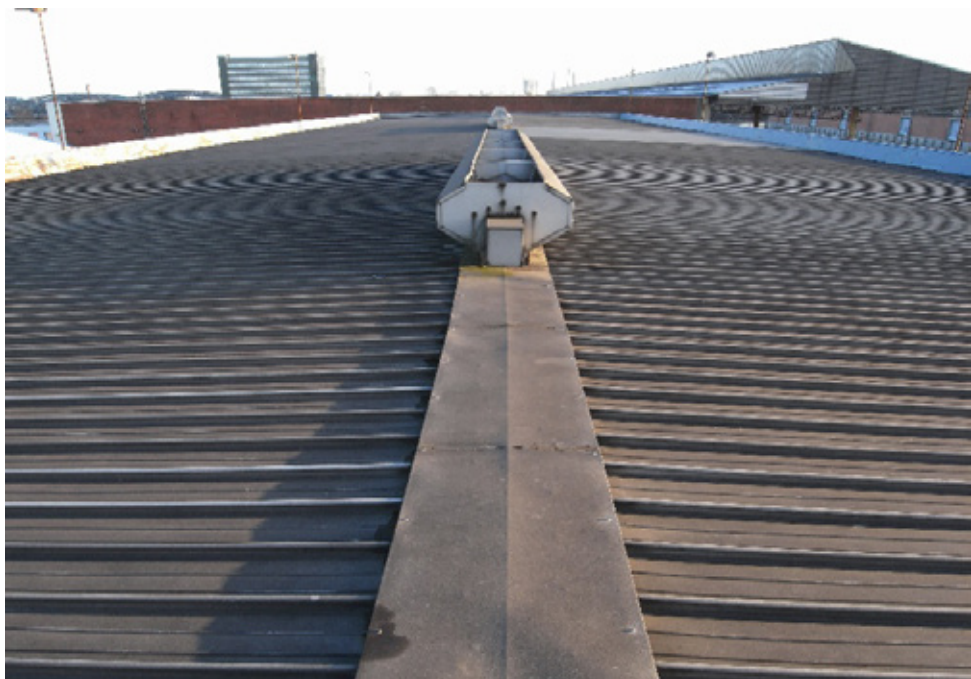
Fig 3.92 Kalzip aluminium roof of the Packing Hall of the Schumacherwerder Overseas Centre, Hamburg
