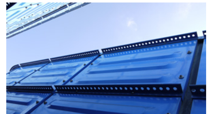
Fig 5.35 Detail of the light blue ribbed cladding of the south façade: note that this is almost the original blue as it has been sheltered from the sun by the pod opposite
