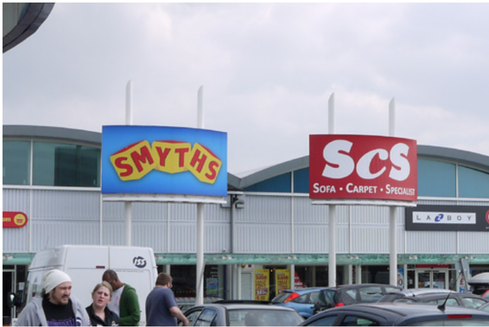
Fig 5.67 Cribbs Causeway Building B Front elevation: polyester powder-coated pressed aluminium panels in a curtain-wall system
