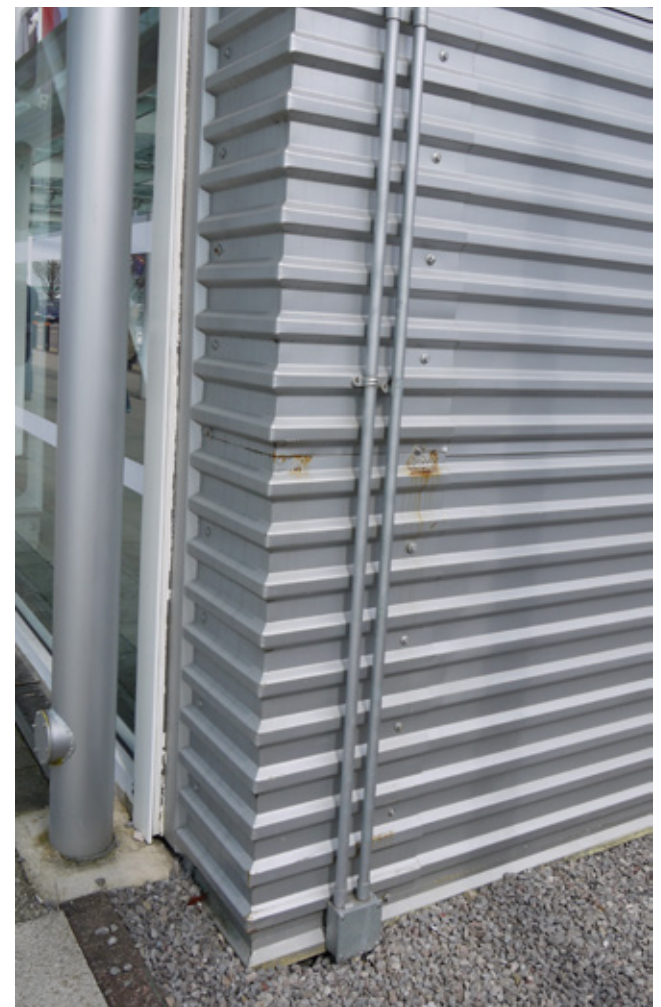
Fig 5.62 Corrosion at the seam detail of the silver PVDF coil-coated steel sheeting
