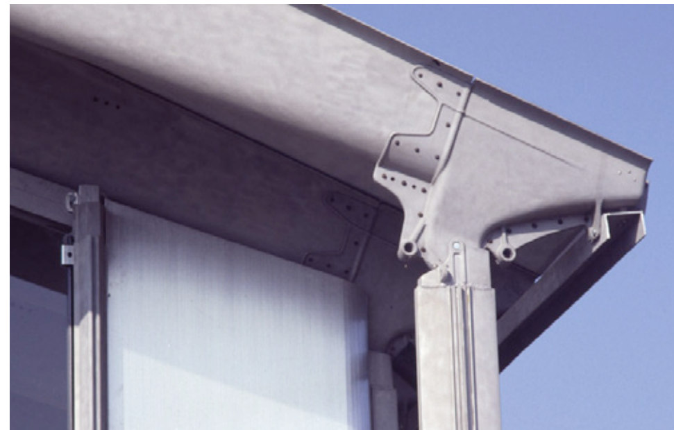
Fig 3.52 Cast aluminium junction between the extruded mullion and fabricated gutter beam of the Aluminium Centenary Pavilion
