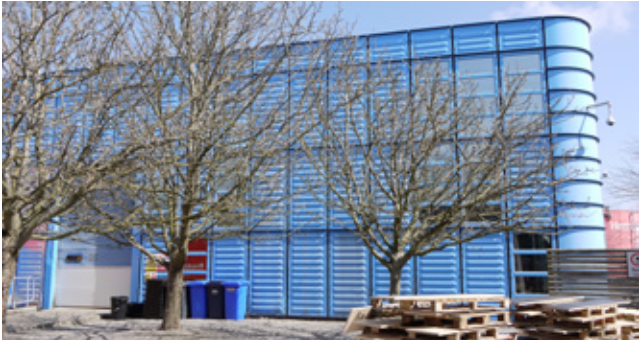
Fig 5.30 The light blue polyester powder-coated aluminium cladding of the west façade has faded and chalked over the course of more than 30 years in the sun
