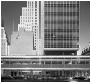
Fig 3.35 Lever House, New York: view from Park Avenue, east elevation – extreme lightweight construction emphasised by the set-back of upper floors and separation of horizontal slab and vertical tower
