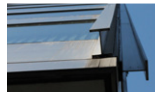
Fig 3.71– Fig 3.72 [above] External details of the articulated aluminium curtain walling, photographed in December 2013
