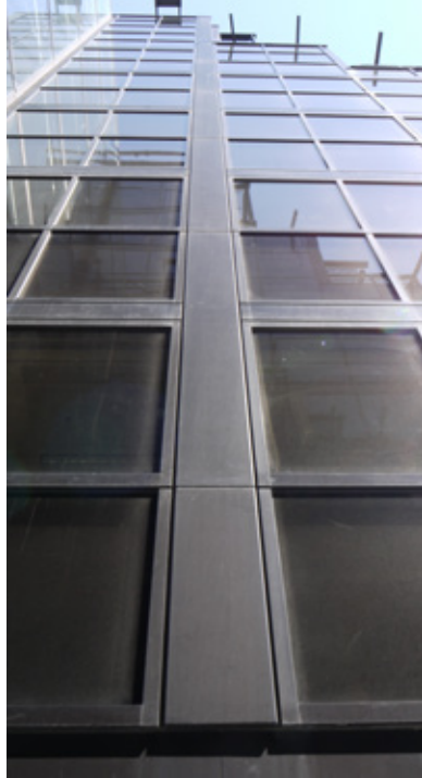
Fig 5.43 [below] The only noticeable weathering of the curtain walling is below certain details and especially at cut ends of extruded sections
