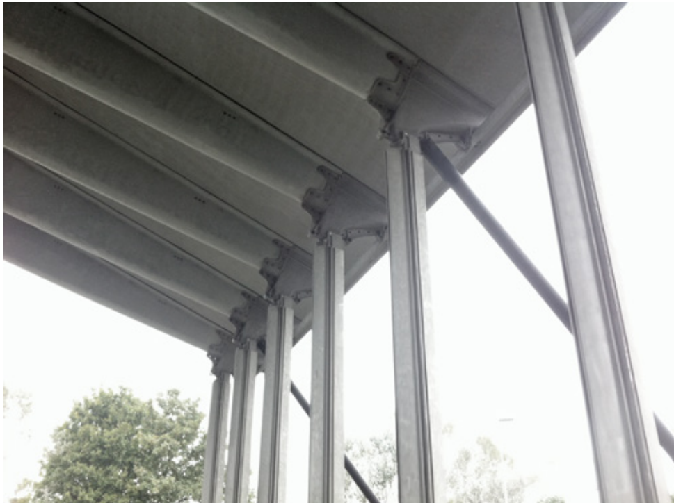
Fig 4.34 Cast aluminium brackets unite beams and extruded aluminium mullions
