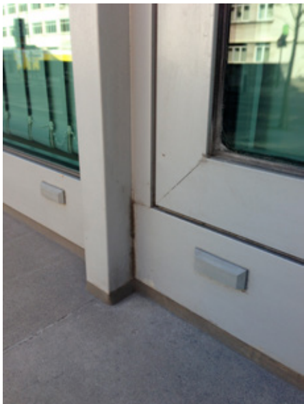
Fig 5.12 Detail of a polyester powder-coated aluminium window
