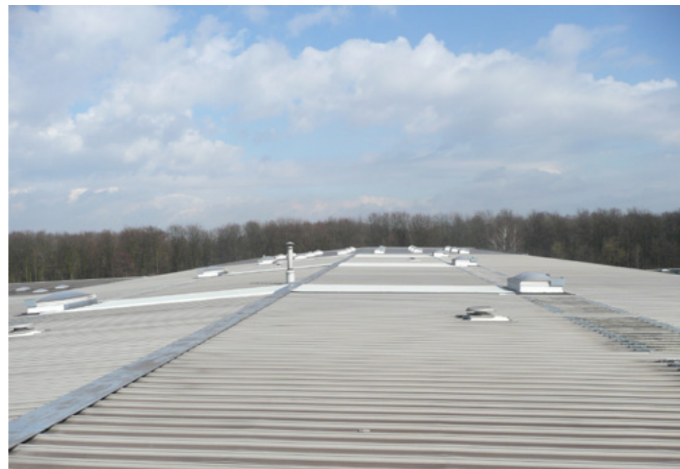
Fig 3.93 Kalzip aluminium roof of the Storage Facility, Essen
