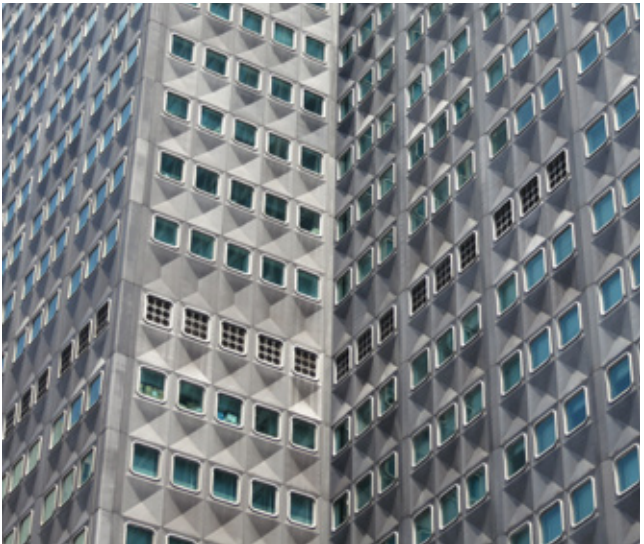
Fig 3.47 Detail view, of the unitised aluminium curtain walling, photographed 2013
