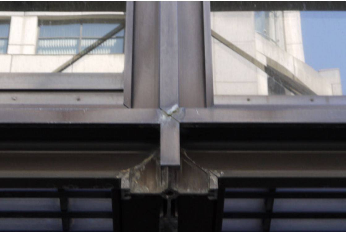
Fig 5.43 [below] The only noticeable weathering of the curtain walling is below certain details and especially at cut ends of extruded sections
