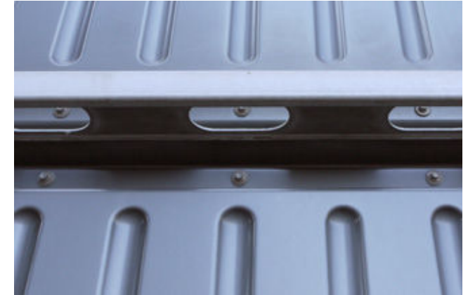
Fig 5.75 Detail of cladding rail and pressed aluminium panels
