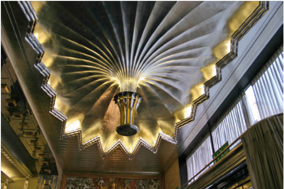
Fig 3.15 Aluminium leaf on the recessed ceiling in the entrance lobby of the Daily Express Building
