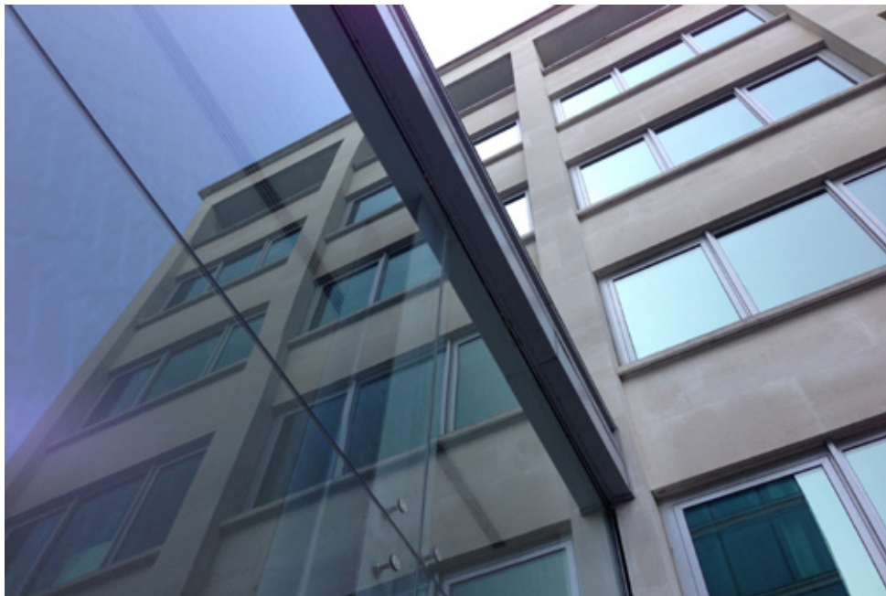
Fig 5.15 Rear extension connection to the original building
