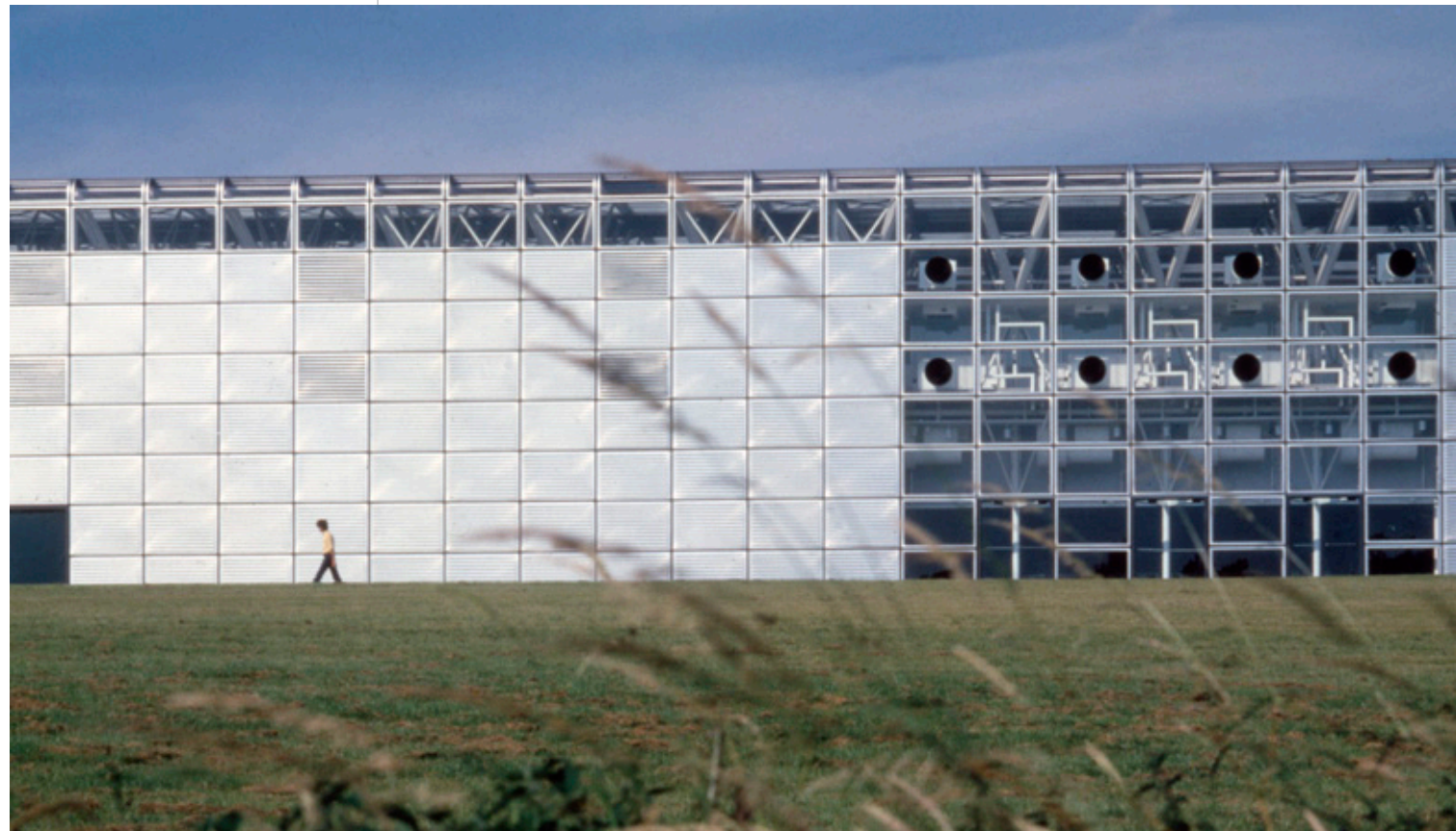
Fig 3.104 Superplastic aluminium cladding and glazing of the Sainsbury Centre for Visual Arts, architect Foster Associates
