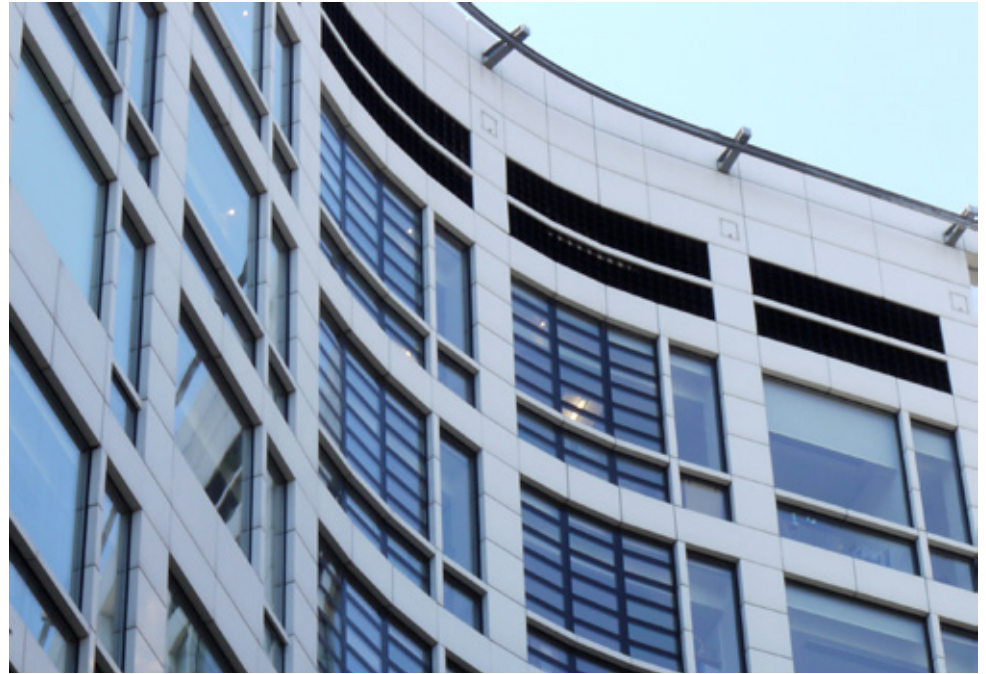
Fig 5.80 New rear façade of Lutyens' House, polyester powder-coated unitised curtain walling, designed by Brookes & Stacey
