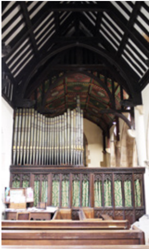
Fig 3.4 Beresford family chapel: aluminium ceiling panels fitted in 1895 and organ installed in 1879
