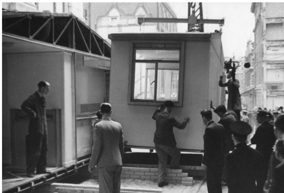
Fig 3.24 Second segment of an AIROH aluminium bungalow being craned into position on brick foundations at the aluminium From War to Peace exhibition on 21 June 1945
