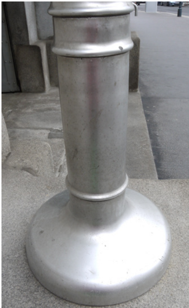
Fig 4.26 [above] The aluminium cladding has wrinkled at the base of one entrance canopy column
