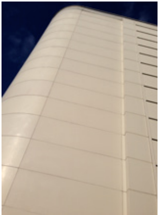
Fig 5.83 Polyester powder-coated aluminium stair tower cladding
