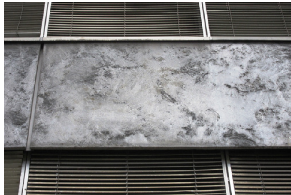
Fig 3.96 Detail of cast aluminium cladding panels, photographed 2013
