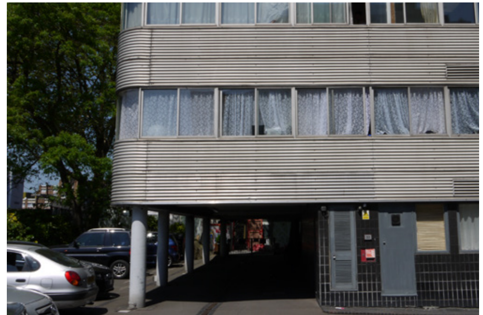
Fig 5.9 Silver anodised aluminium ribbon windows and cladding
