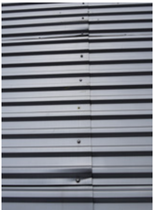
Fig 5.64 Silver PVDF coil-coated steel sheeting of Cribbs Causeway, note poor original workmanship remains dissatisfactory for the life of a building, unless remedial work is undertaken
