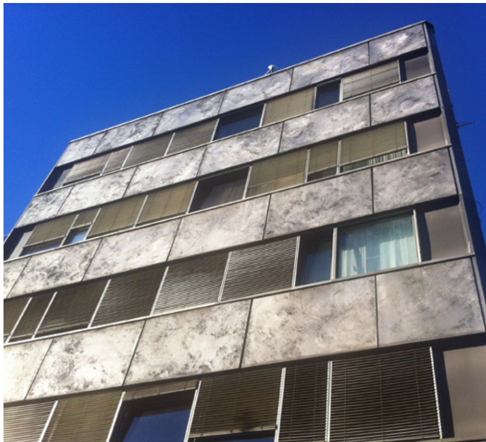
Fig 3.94 Cast aluminium cladding panels creating a stone effect on the façade of the Television Centre, Ljubljana, photographed 2013
