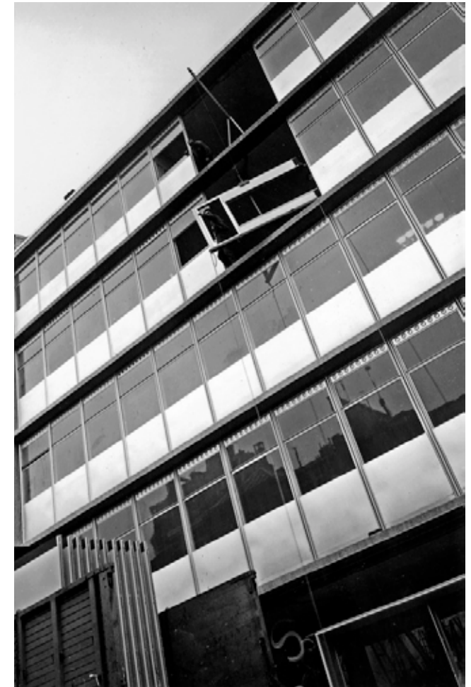
Fig 3.27 Unitised aluminium curtain walling being installed on Fédération Nationale du Bâtiment Offices, Paris
