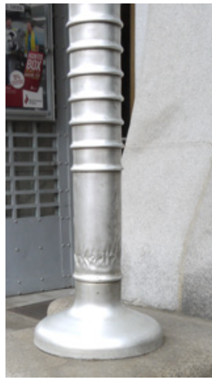
Fig 4.26 [above] The aluminium cladding has wrinkled at the base of one entrance canopy column
