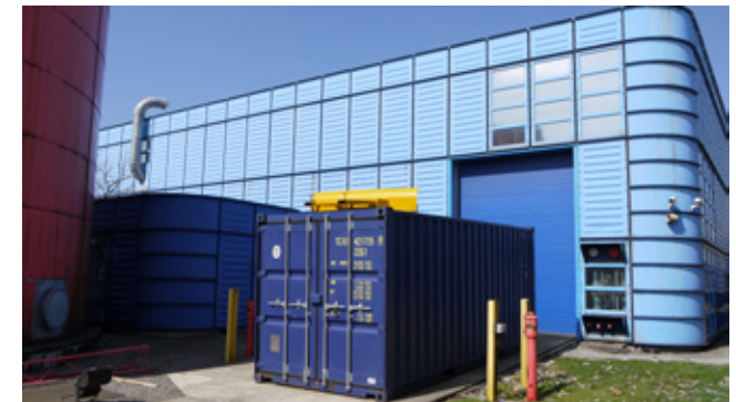
Fig 5.33 Polyester powder-coated pressed aluminium: note the new shutter door
