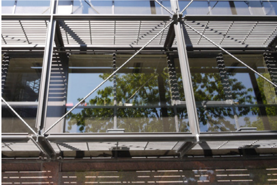
Fig 5.39 Bronze anodised curtain walling of 1 Finsbury Avenue
