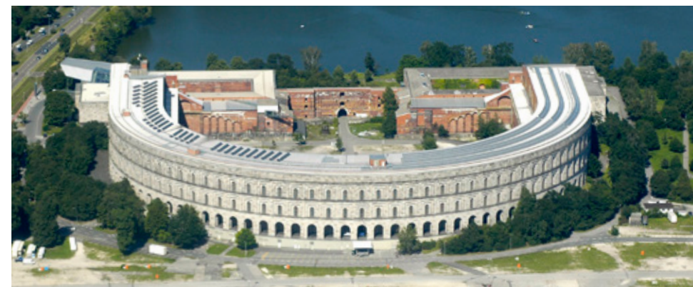
Fig 3.89 Aerial view of Kalzip's profiled aluminium standing seam roof of the Nuremberg Congress Hall, installed in 1968
