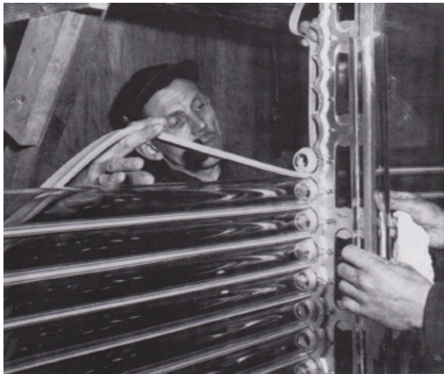
Fig 3.28 Johnson Wax Research Tower: tubular glazing system, 1939
