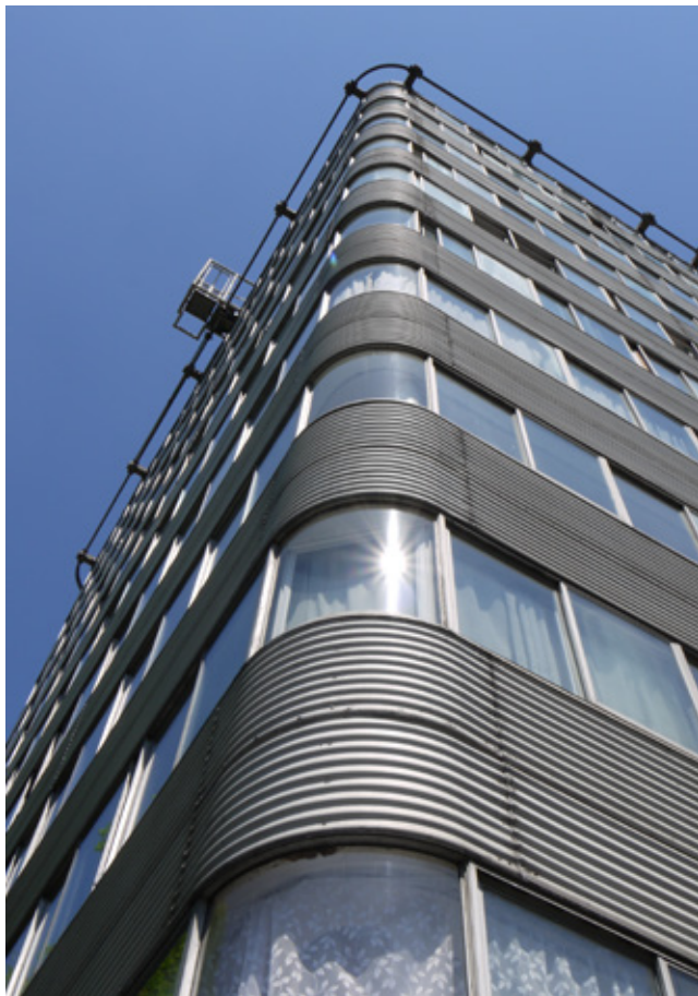
Fig 5.8 Curved corner of 125 Park Road: note the cleaning access system
