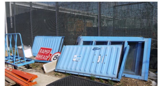
Fig 5.34 Spare interchangeable polyester powder-coated pressed aluminium panels and windows – a result of the newly installed shutter door
