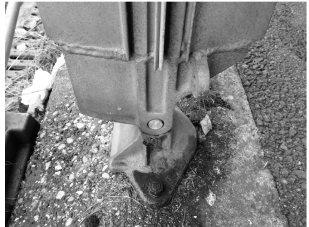
Fig 4.37 Cast aluminium footings of the Aluminium Centenary Pavilion
