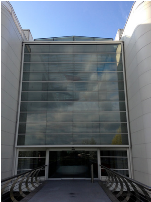
Fig 5.86 Polyester powder-coated aluminium corner panels
