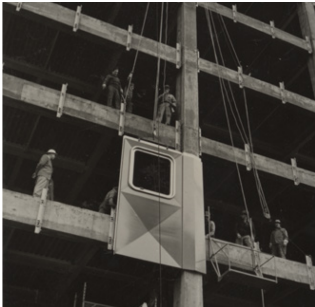
Fig 3.49 The first unitised curtain-walling panel being installed on the Alcoa Building. The panels are secured to flanged fittings bolted to fire-proofed steel beams.
