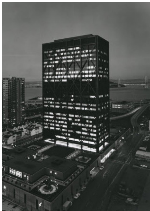
Fig 3.88 The Alcoa Building in San Francisco was constructed as a stiff cage, designed to withstand seismic forces
