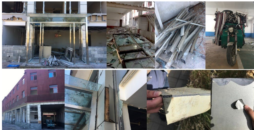
Figure 5-5 Aluminium building parts in the demolished commercial buildings of the Tongzhou district.
