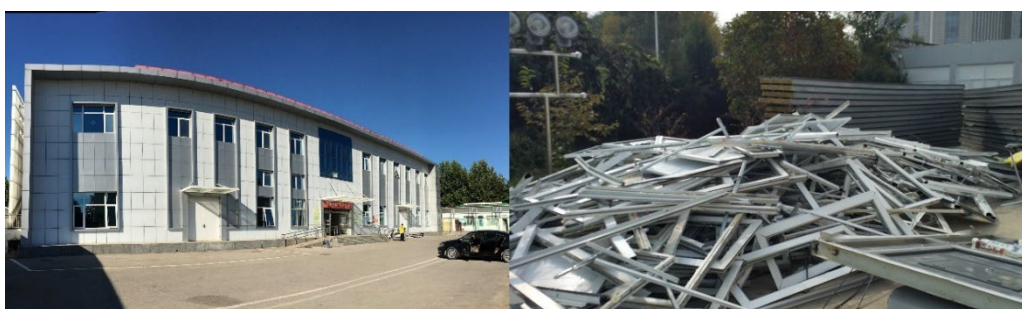
Figure 5-7 Aluminium building parts in the demolished commercial buildings of the Shunyi district.
