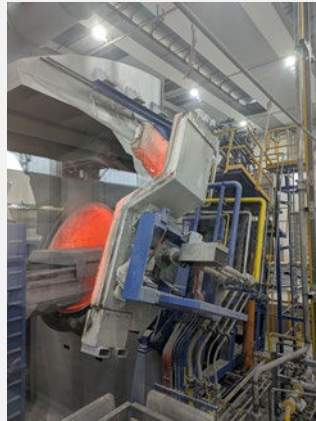
Adding the charge to the preheated furnace.
